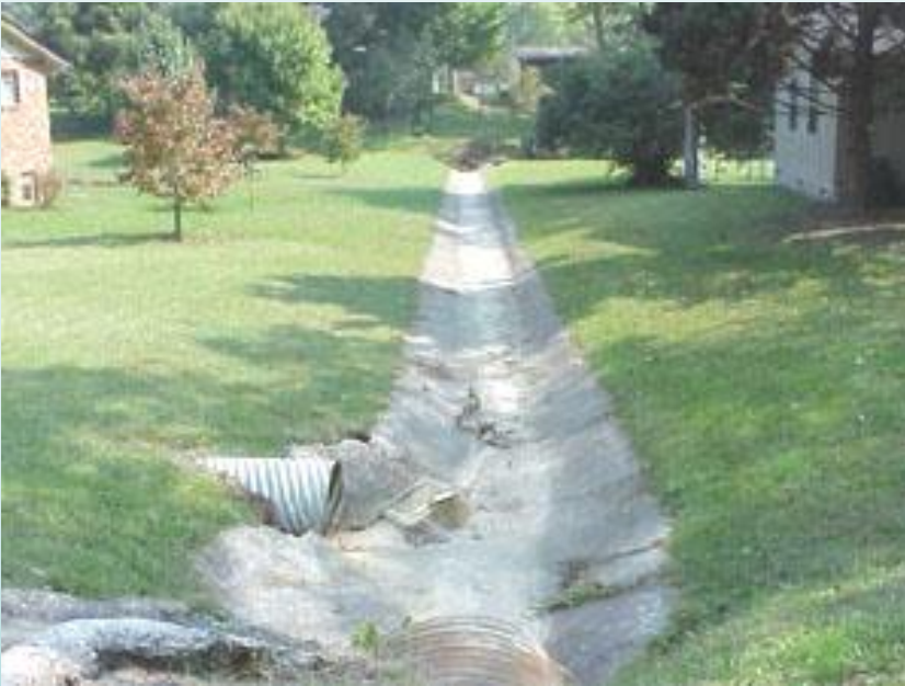
Conventional Concrete-Lined Channel
