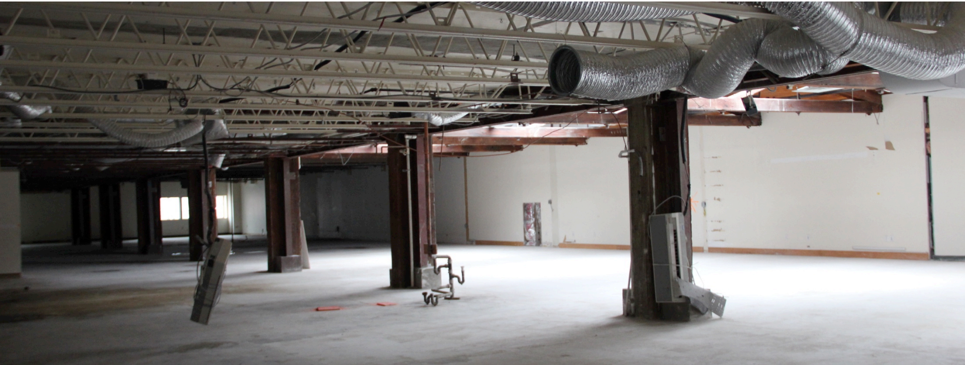
First floor after interior demolition
