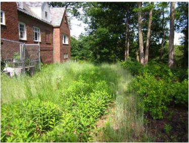
**Figure 3: Bioretention Basin**
