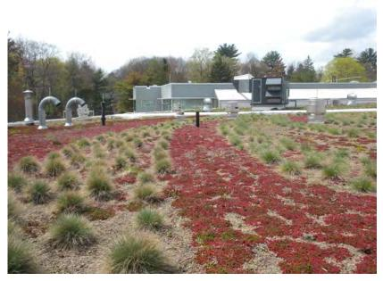
**Figure 8: Extensive Green Roof**
