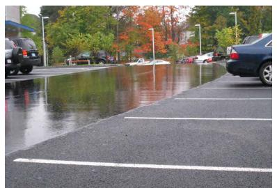
**Figure 7: Porous Asphalt Parking Stalls**
