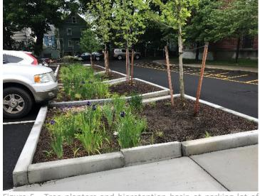
Figure 5. Tree planters and bioretention basin at parking lot of Irving School in Roslindale, Boston. [Source: Boston Water and Sewer Commission (BWSC) and Greenovate City of Boston]
