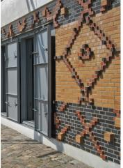
Figure 2a. Flood Protection Shutters [Source: City of Hamburg, Germany]
