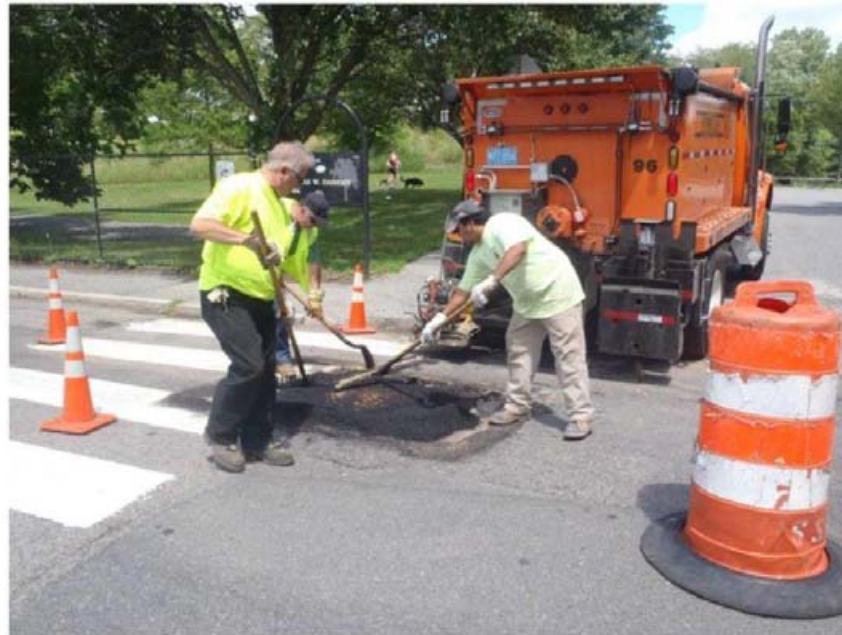
(L): The Street Maintenance Division repairs a pothole near Danehy Park. (R): Maintenance operations serve to reduce emergency back-ups and flooding.
