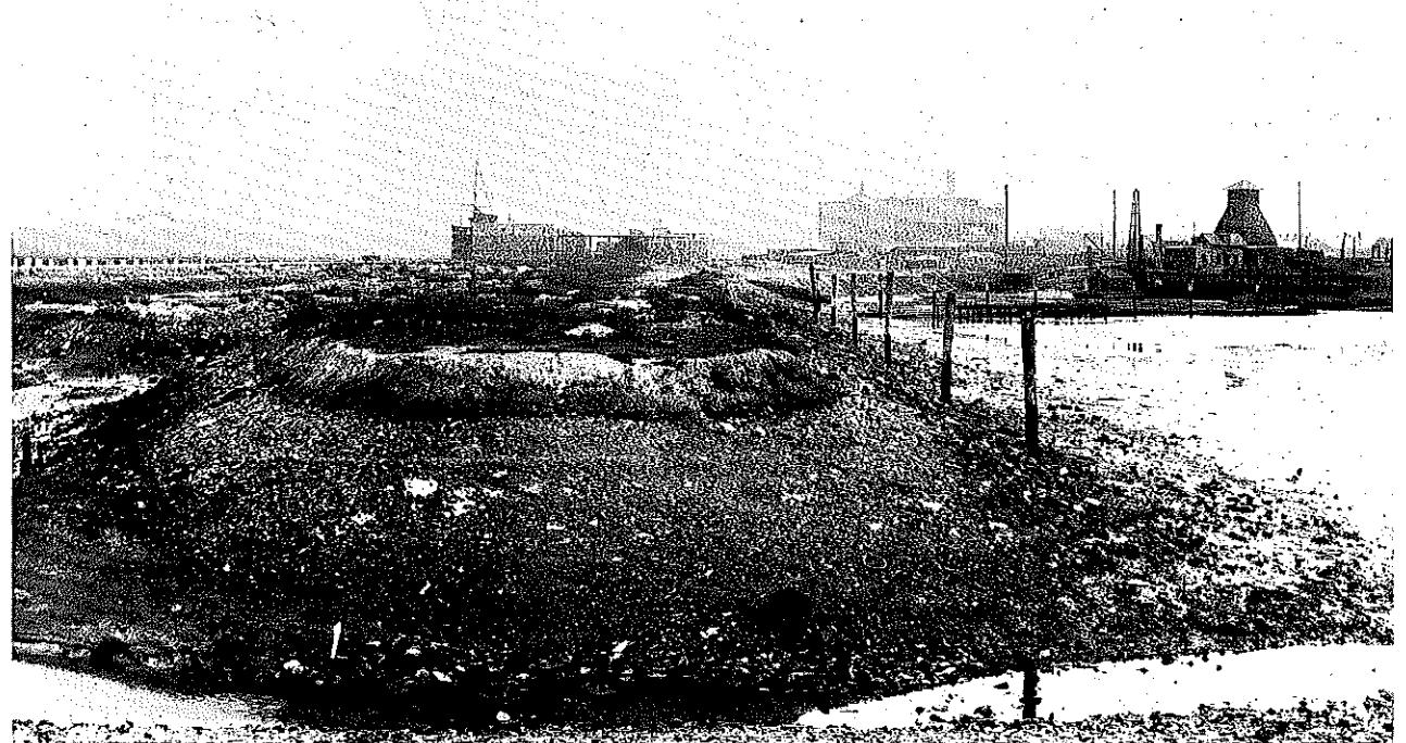
45. Fill in place for Commercial Avenue, from the north side of the Lechmere Canal, 1900 3059
