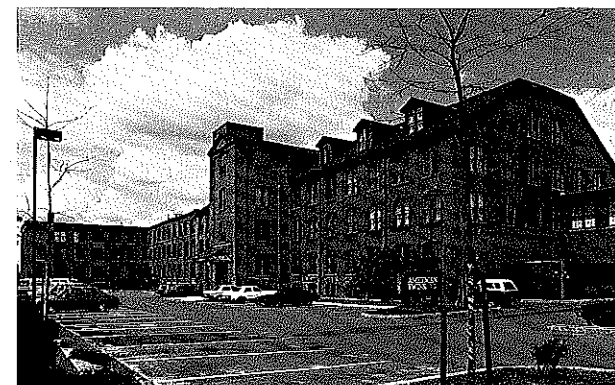
80. American Twine Office Park, 222 Third Street, 1875, original architect unknown. Renovation by Sutphin, Morris & Associates, 1982
