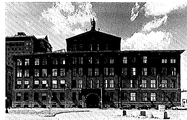
78. Athenaeum House, 215 First Street, 1895, Lockwood, Greene & Company. Renovation by Symmes, Maini & McKee, 1979-83 4857
