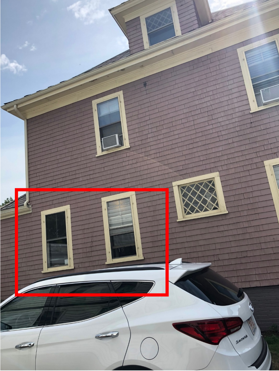
ALTERNATE VIEW OF TWO WINDOWS TO BE REPLACED (LEFT, FIRST FLOOR)
