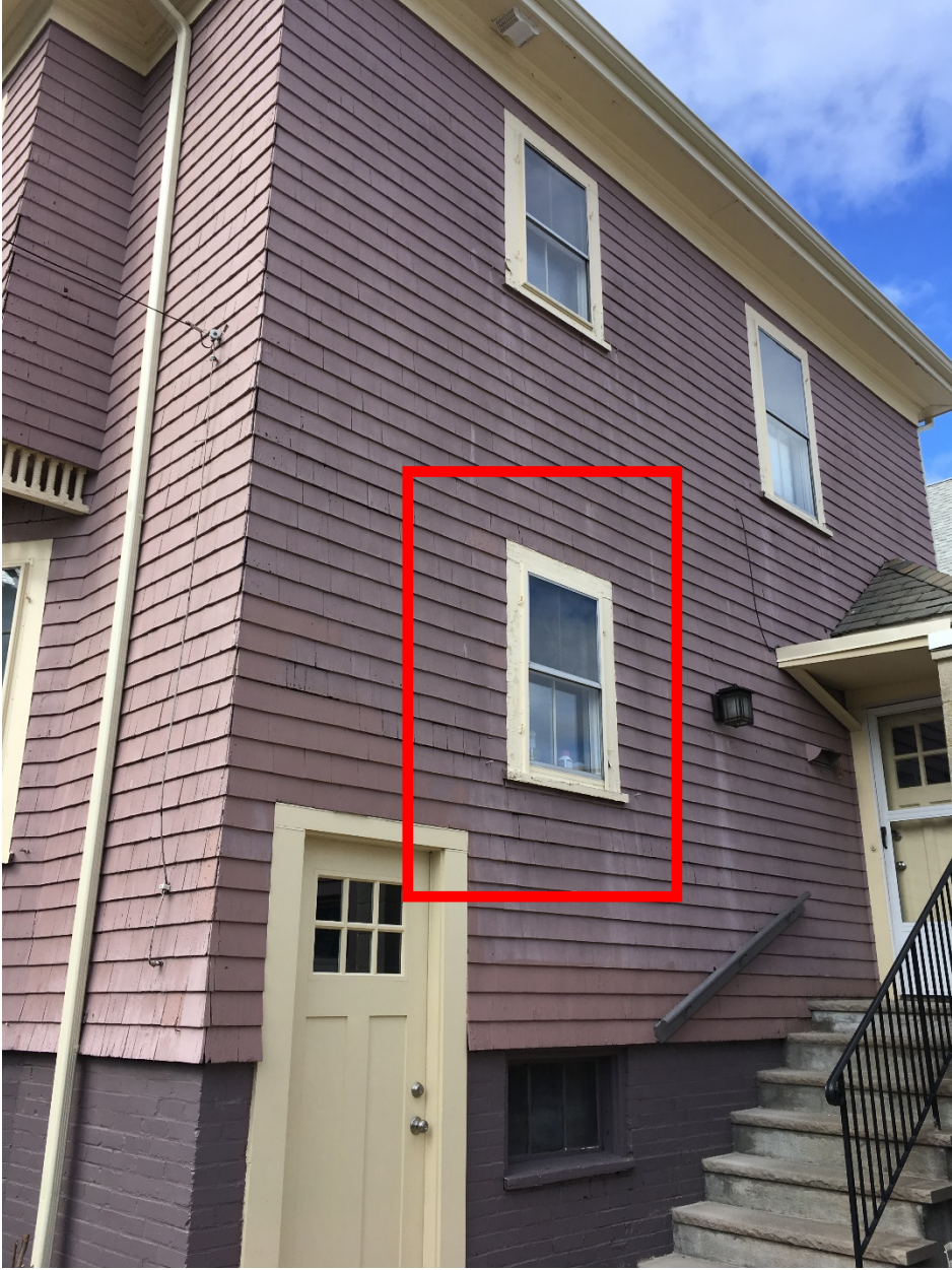
ADDITIONAL VIEW OF SOUTH FAÇADE & WINDOW TO BE REPLACED.
