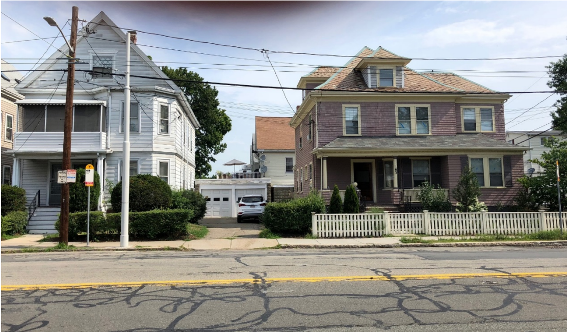
VIEW OF 103 BELMONT (RIGHT) AND 105/107 BELMONT (NEIGHBOR, LEFT) GARAGES OF BOTH PROPERTIES CAN BE SEEN. GARAGE OF NEIGHBOR FACES STREET
