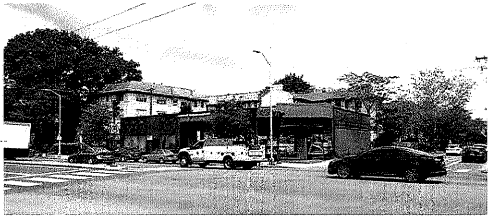
04 View of existing building across Mass Ave.
