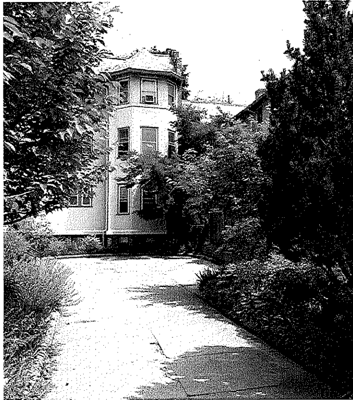
09 View of 1617, 1619 Mass Ave. entry
