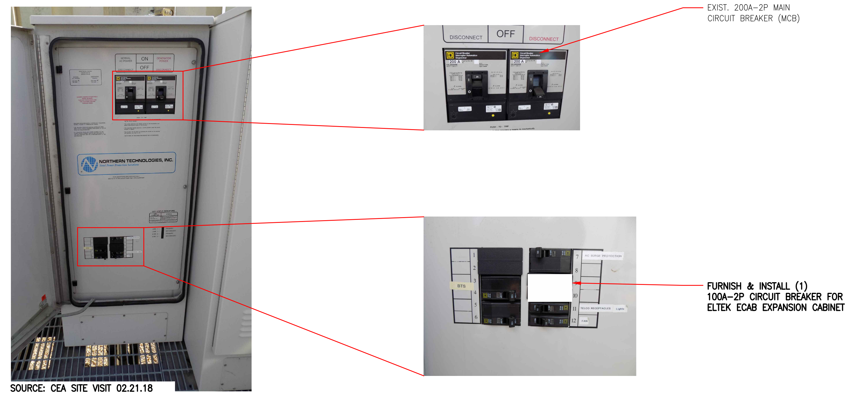
EXIST. PPC BREAKER PANEL SCALE: NTS 2 E-1
