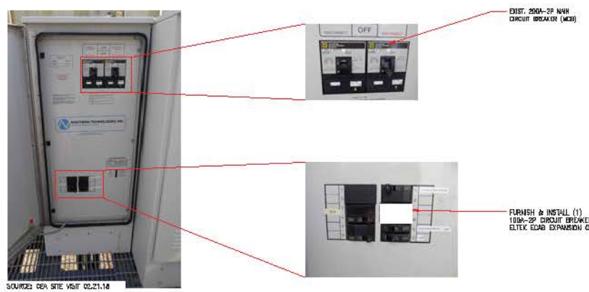
EXIST. PPC BREAKER PANEL SCALE: NTS
