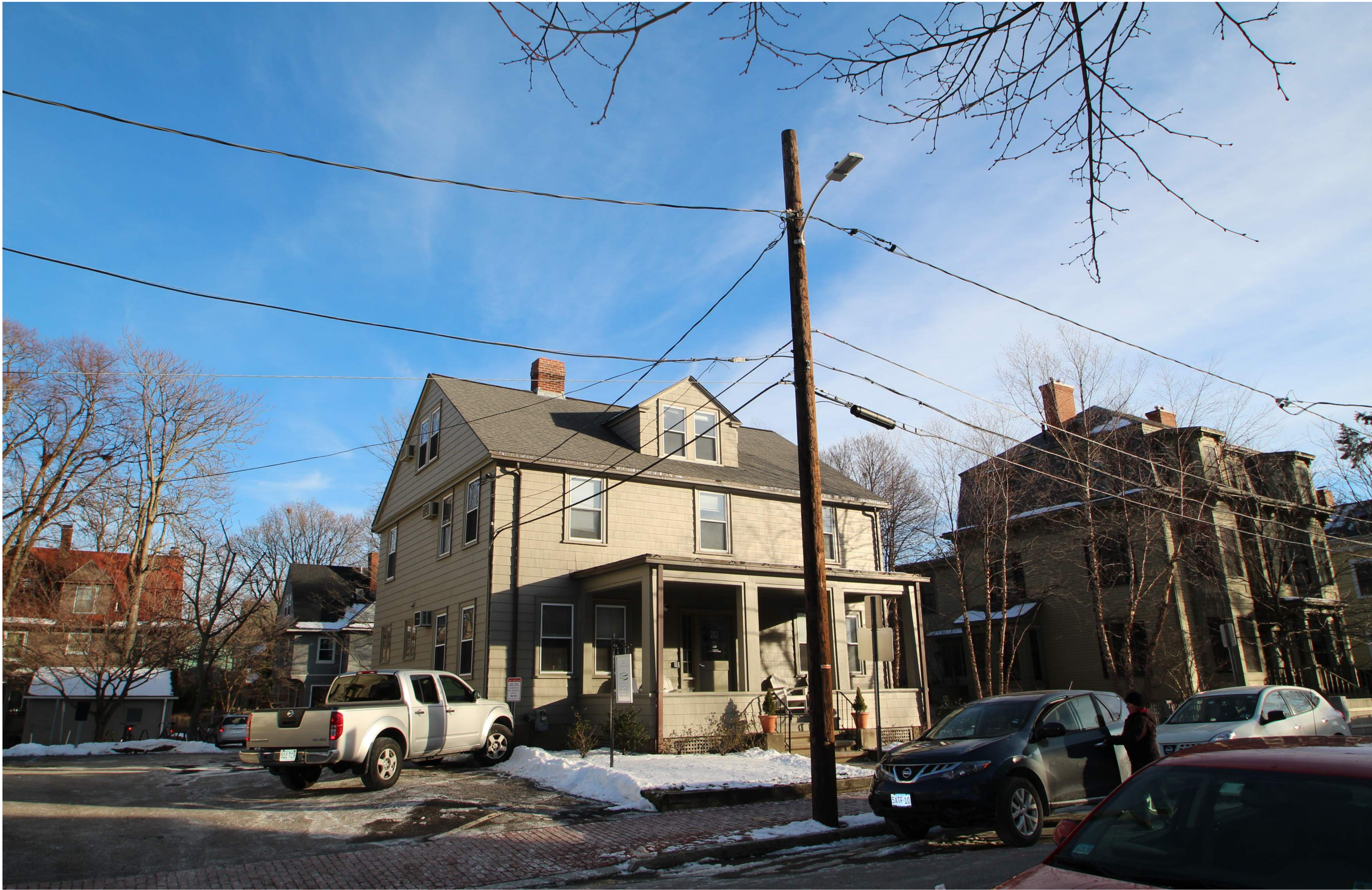
Front (West) & Side (North) Facades
