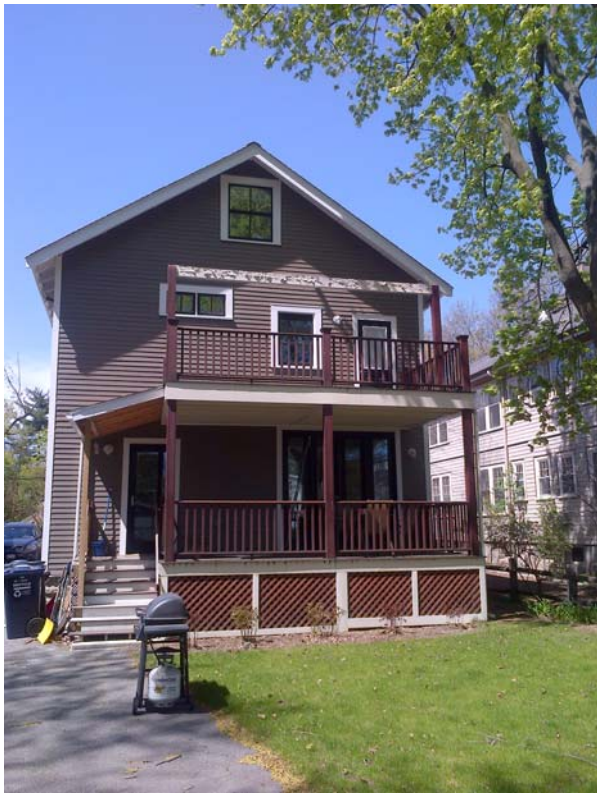
REAR FAÇADE OF HOUSE
