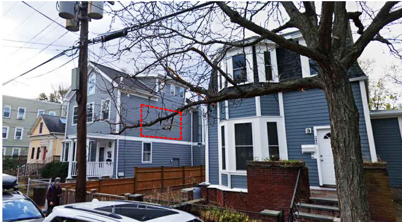
EXISTING PHOTO FRONT RIGHT
