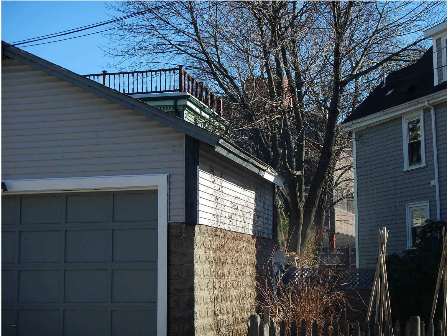
VIEW SOUTHEAST FROM COTTAGE PARK AVENUE (EQUIPMENT NOT VISIBLE)
