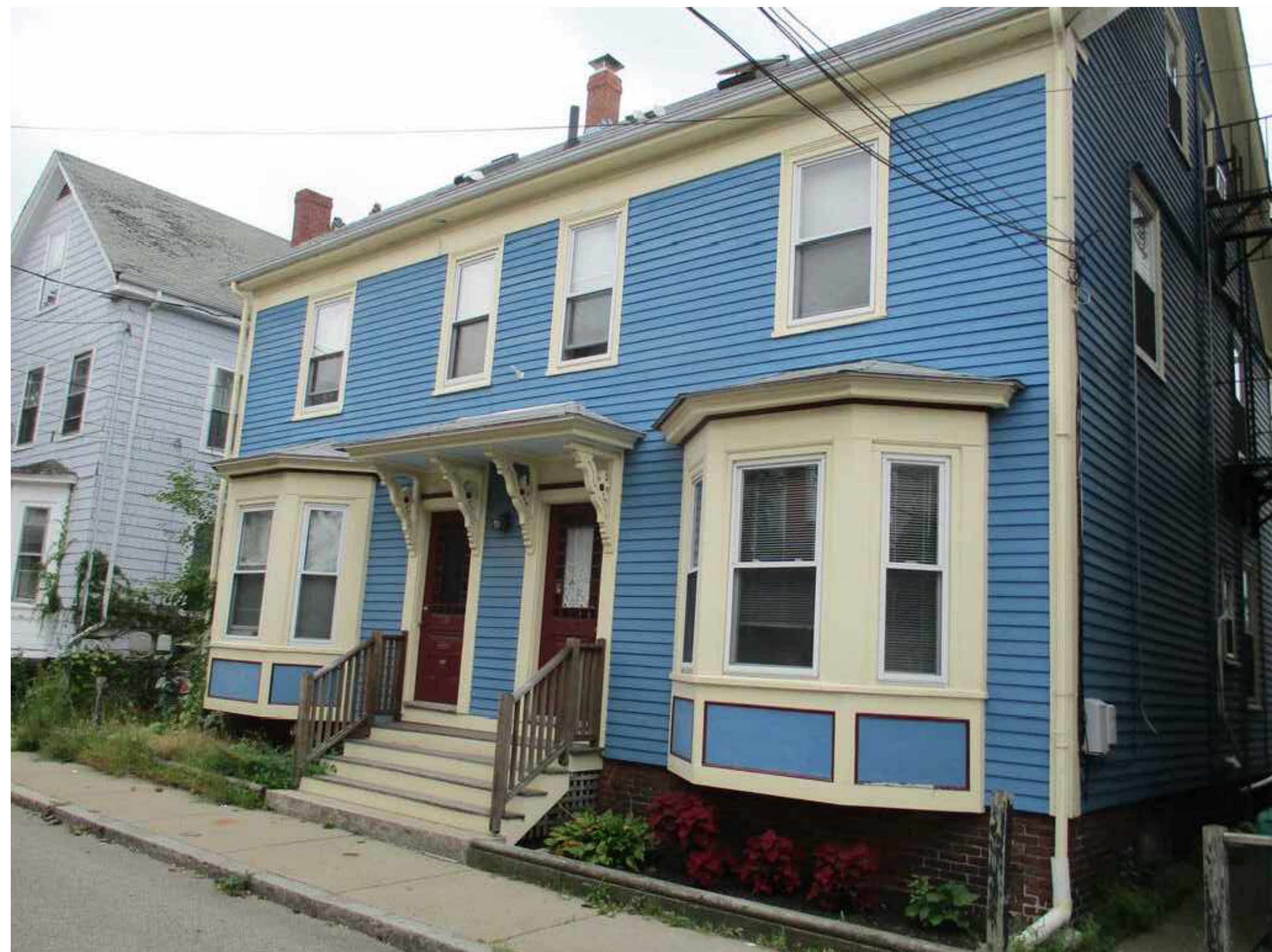
0-2 FAIRMONT AVE STREET VIEW - NO CHANGE
