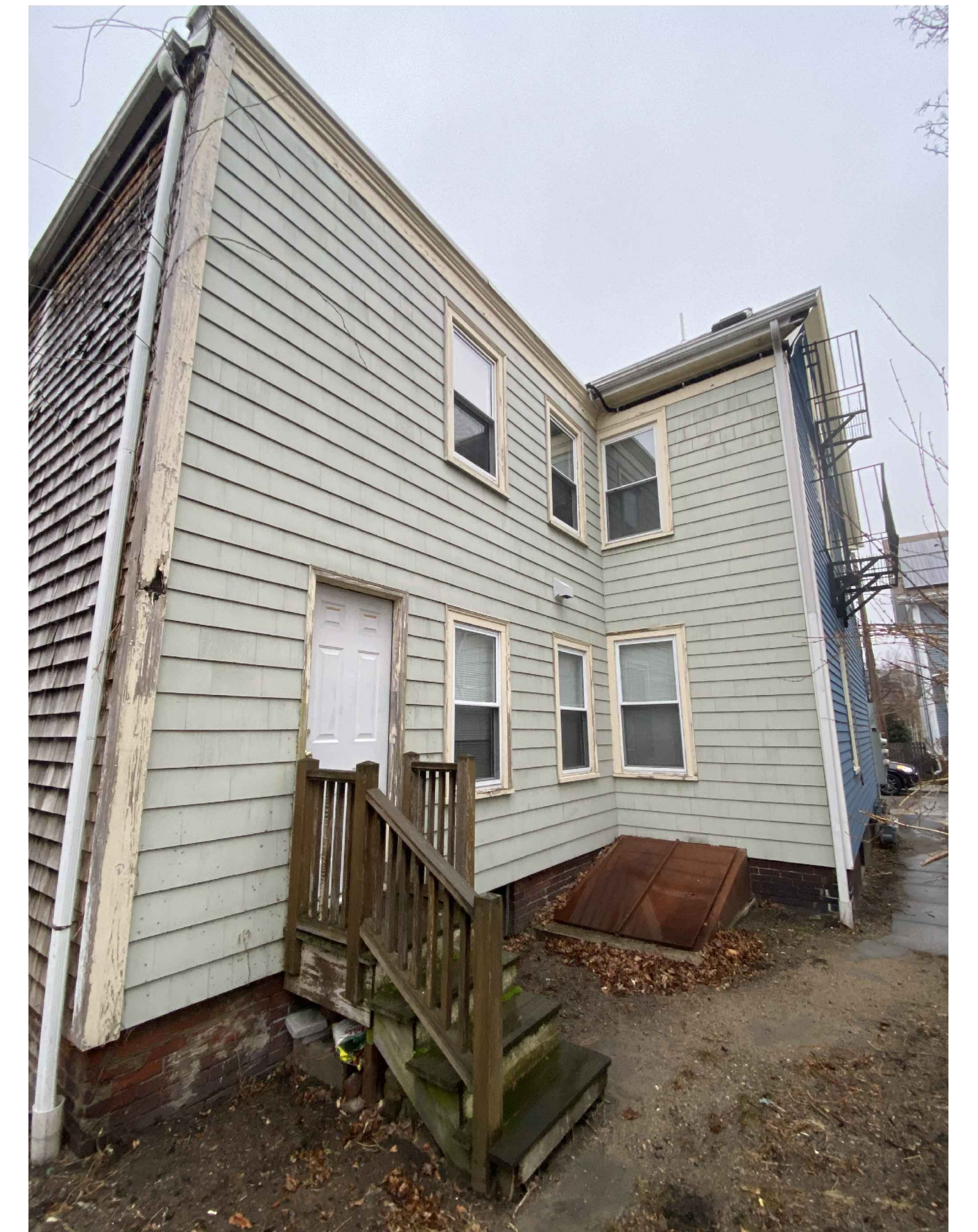
VIEW OF REAR FACI BULKHEAD AND LEFT SIDE ENTRY
