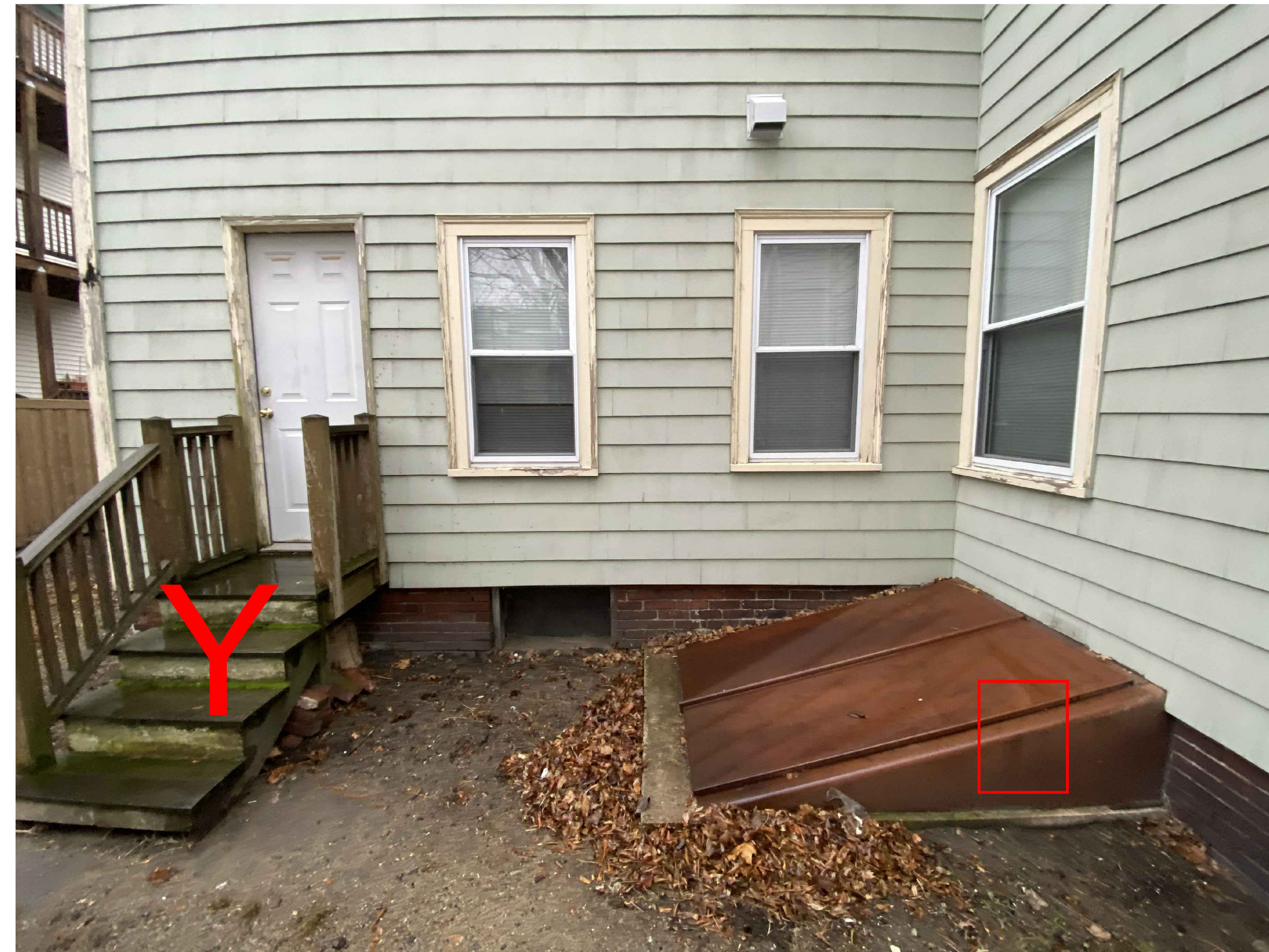
VIEW OF REAR FACI BULKHEAD AND LEFT SIDE ENTRY
