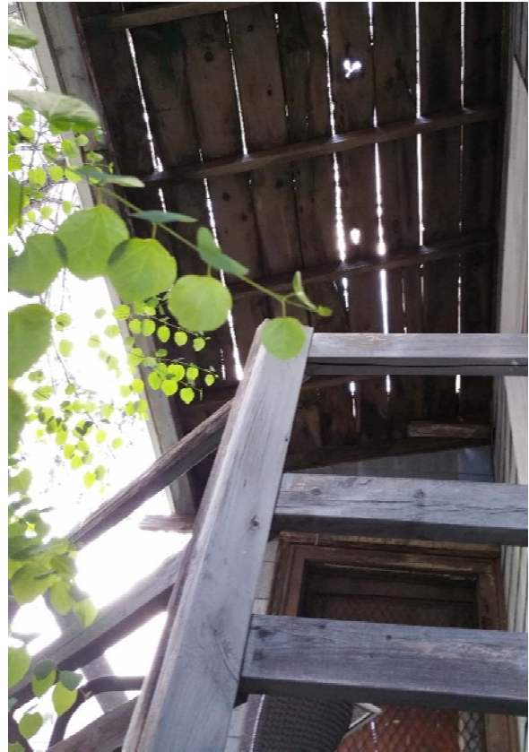
Existing rear porch as seen from existing rear stairwell to basement
