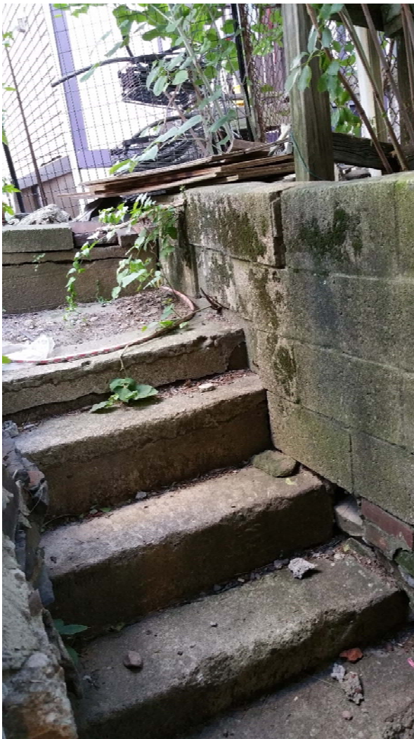
Existing concrete stairs from rear basement door
