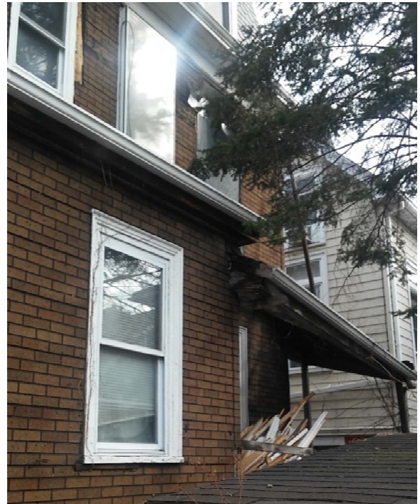
Existing rear porch roof as seen from neighbor's driveway (looking northeast)
