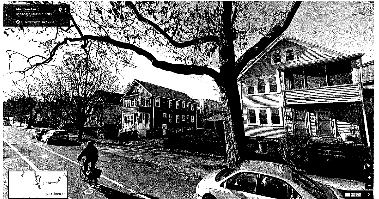
38-40 ABERDEEN AVENUE - STREET VIEW FROM NORTHEAST
