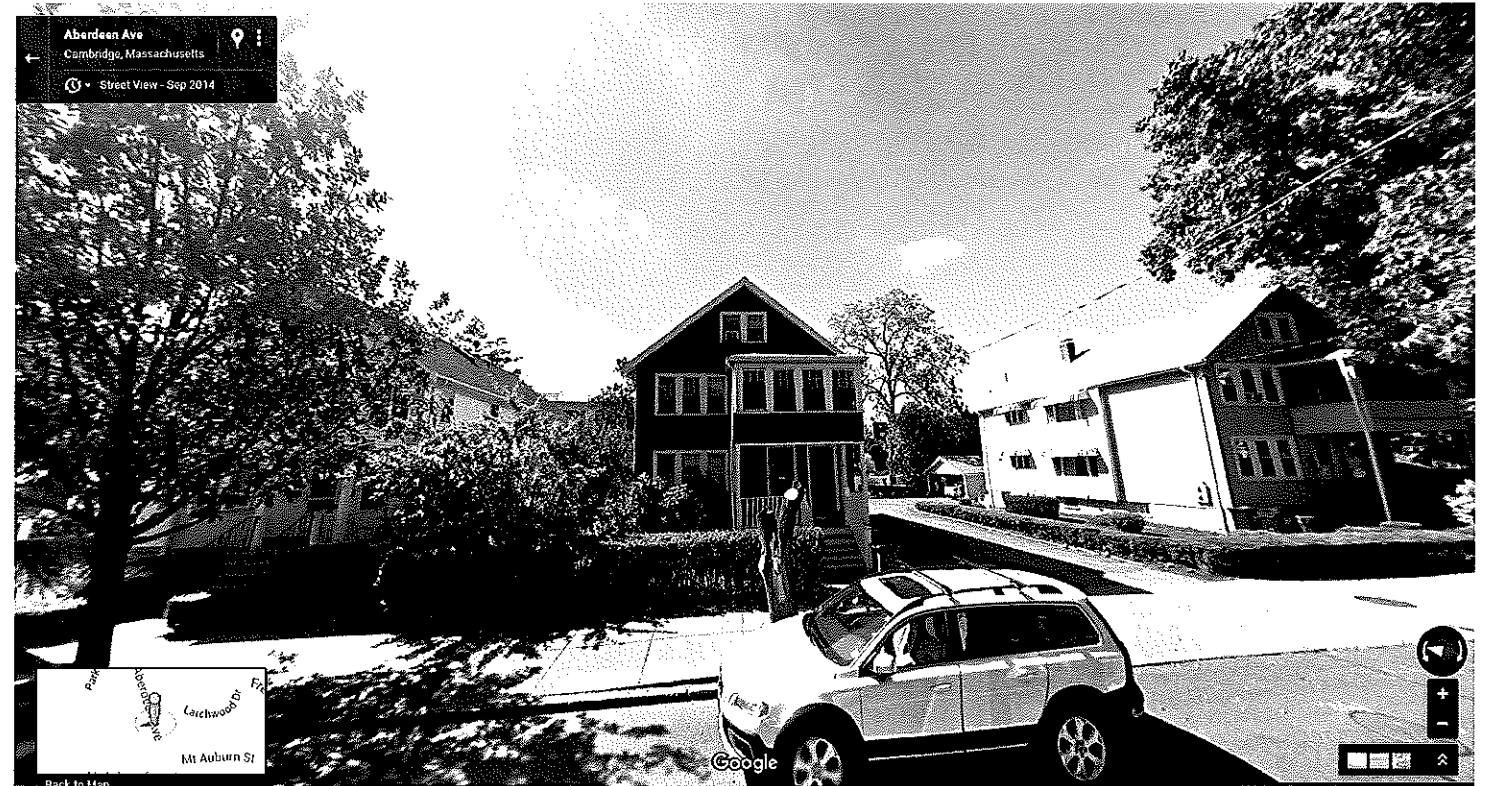
38-40 ABERDEEN AVENUE - STREET VIEW FROM EAST
