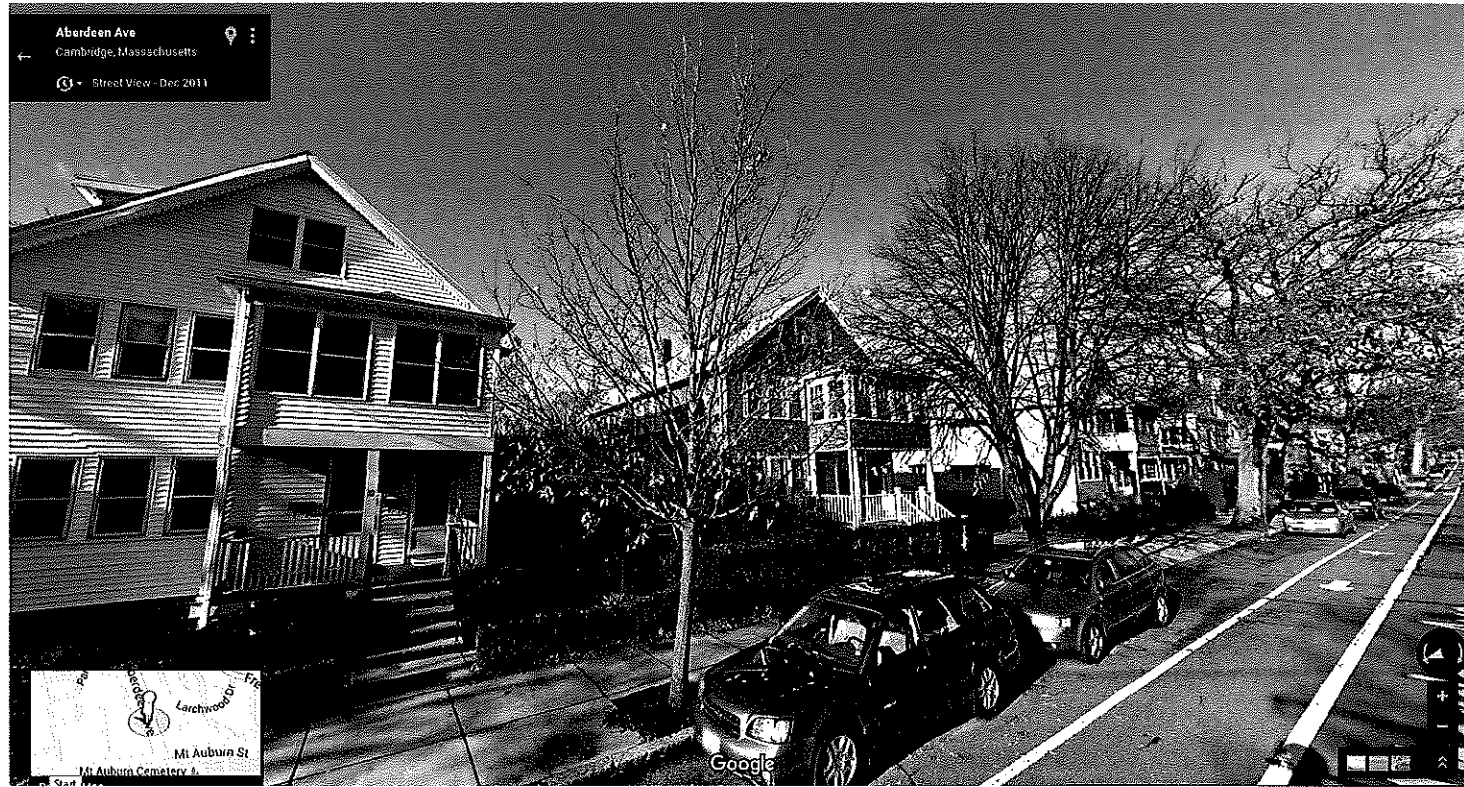
38-40 ABERDEEN AVENUE - STREET VIEW FROM SOUTHEAST
