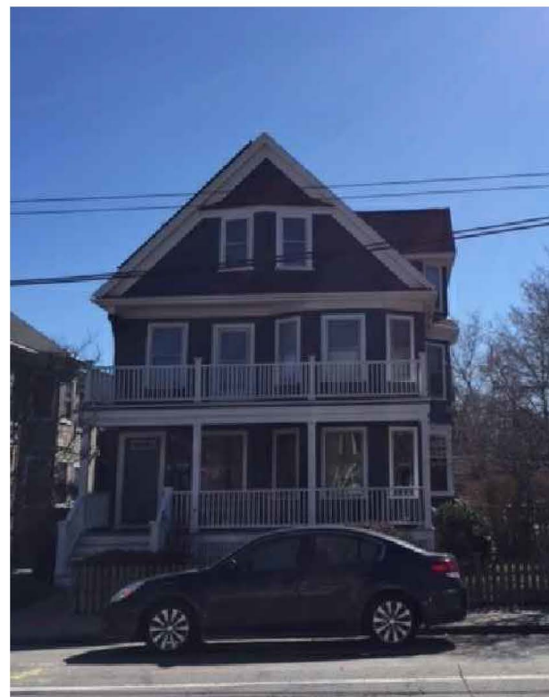
5 FRONT VIEW 486 HURON AVENUE
