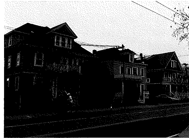
2 STREET VIEW (WEST) 478 TO 486 HURON AVENUE
