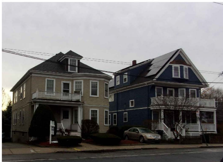
4 FRONT VIEW (WEST) 482 TO 486 HURON AVENUE
