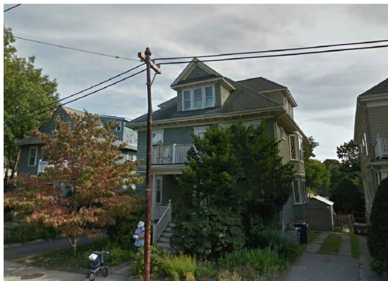
1 FRONT VIEW 478 HURON AVENUE
