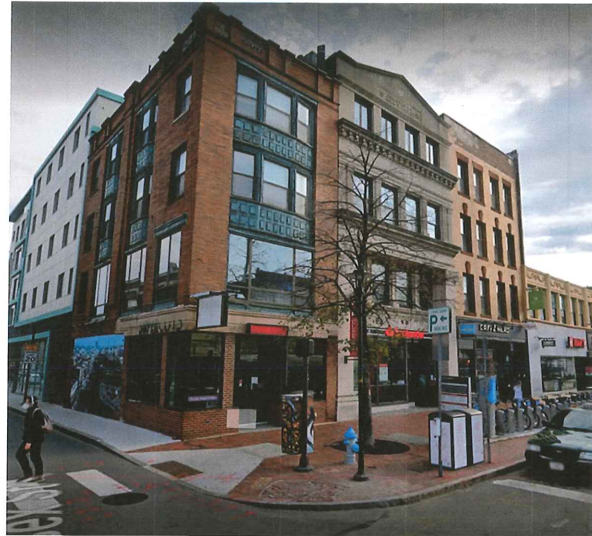
Existing View of Property
