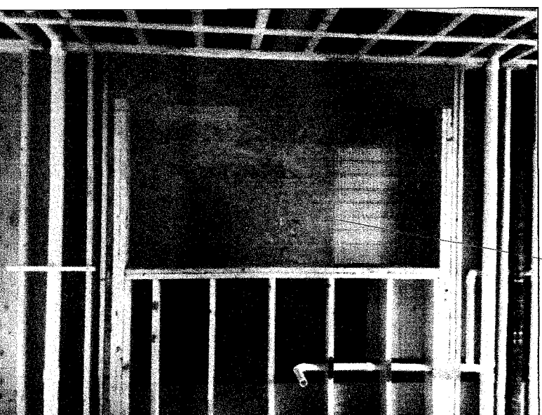
INTERIOR FRAMING FOR NEW BAY WINDOW
