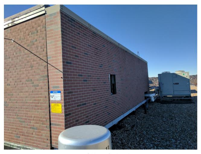
Figure 6: View of alpha sector fiberglass enclosure
