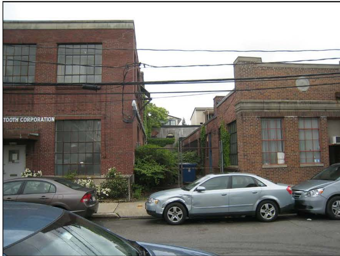
○ SOUTH FACADE & EAST ALLEY
