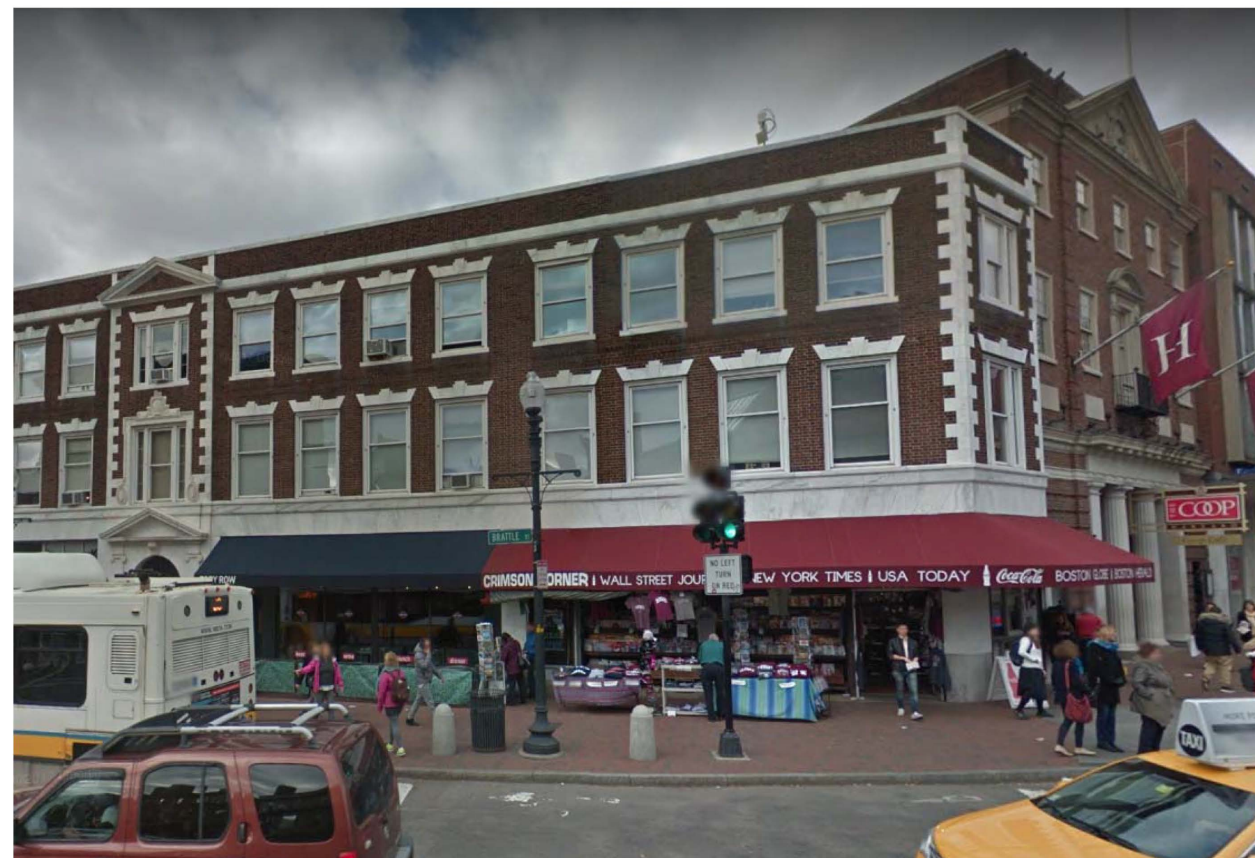
EXISTING EXTERIOR FACADE
