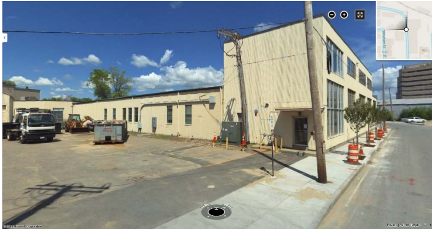
View of site looking North
