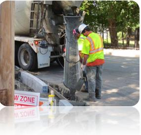
reset, crews will pour the new concrete sidewalks, followed by any brick work that remains.
