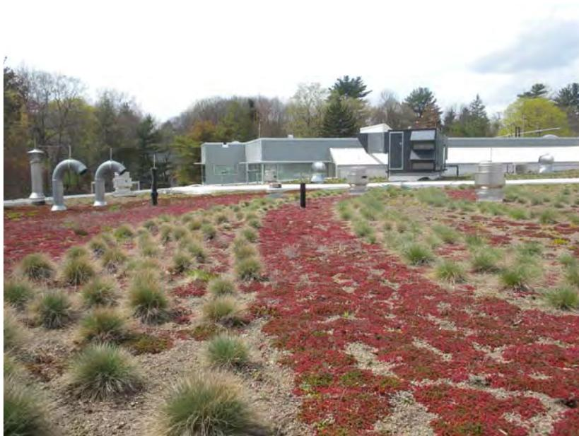
**Figure 8: Extensive Green Roof**
