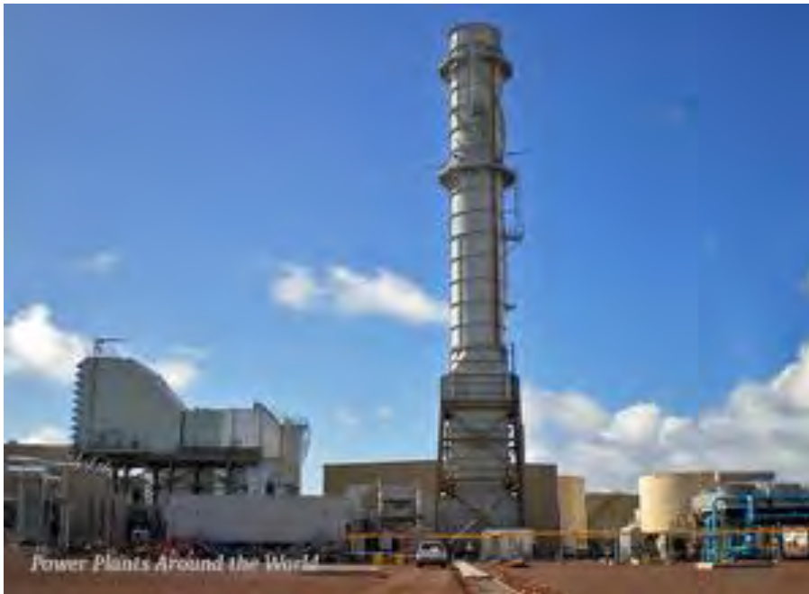
Natural Gas Plant http://www.industcards.com/cc-usa-hi.htm
