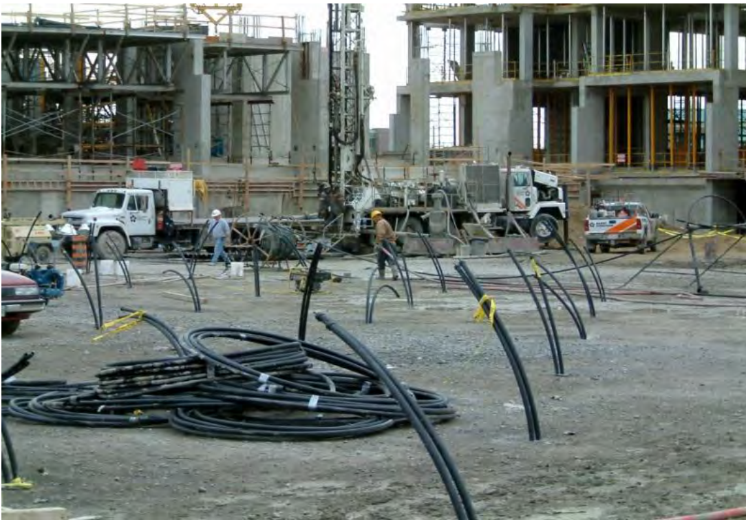
Installation of a Geothermal System (Integral Group)
