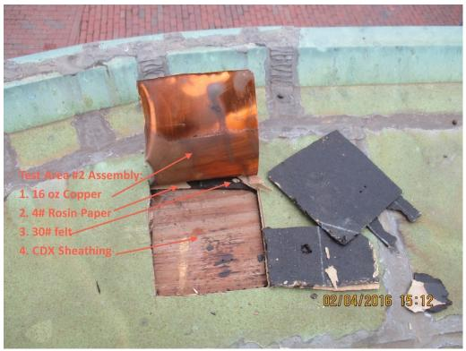
Photo 19 North elevation: Test Area #2 assembly.
