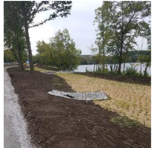
A bio-swale permitted by the Conservation Commission and installed as part of the Fresh Pond Drainage and Community Garden Project.
