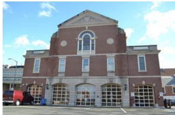
Built in 1934, Fire Headquarters houses Fire Administration, Engine One, Ladder One, Rescue One, Hazmat One, the Dive Rescue vehicle, and the Division Three SUV.
