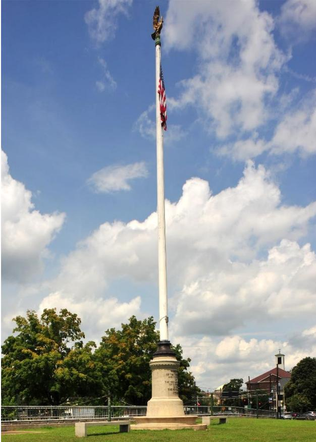
The Revolutionary memorial flagstaff was installed in 1914. The current pole, which dates from 1930, has been repeatedly shortened as the base rotted. A new pole would be closer to the original height of 100+ feet.
