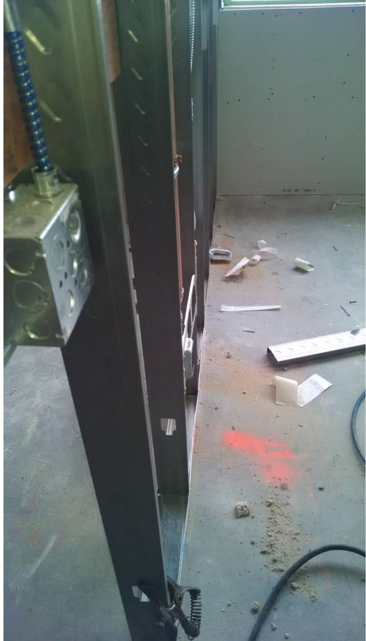
However the same wall viewed from the other side, you see that almost all of the stud bays have some type of obstruction, even electrical and plumbing for the adjoining room, even if it appears as a breachable wall! Out of the five stud bays shown, only one would allow sufficient room for a firefighter, fully geared to crawl through. The bottom line is KEEP TRYING!
