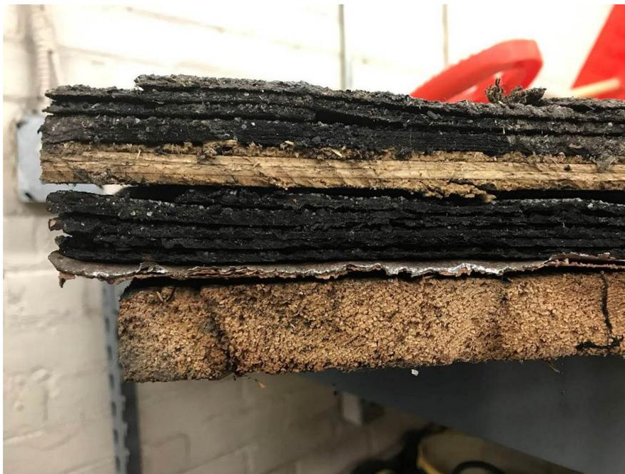
Truck companies are expected to get to the roof and vent but often run into obstacles such as this. Clearly a code violation. This photo is NOT from Cambridge, but could happen anywhere! Starting from the lowest layer – wood roof sheathing, metal roof, 3 layers of asphalt shingles, 1/2" plywood with another 3 layers of asphalt shingles.
