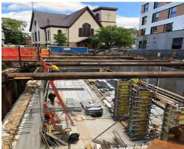
Previous funding supported the construction of a 480,000 gallons stormwater tank in the City's parking lot on Bishop Allen Drive and the jacking of a 60" diameter pipe under the MBTA redline on Mass. Ave. to carry stormwater from the neighborhood to the Charles River.
