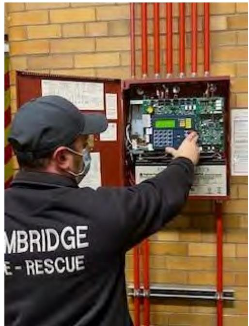
A member of Fire Prevention inspecting/testing a Fire Alarm Control Panel
