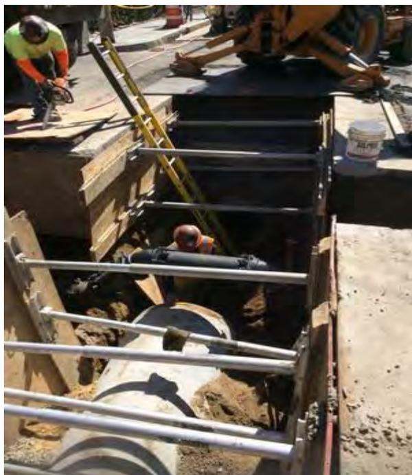
Previous funding was used for emergency repair and replacement of existing infrastructure, such as this section of drain line on Pearl Street (shown left).
