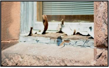
Window sills must be restored or replaced. Storm windows would minimize energy loss and allow retention of original sash.
