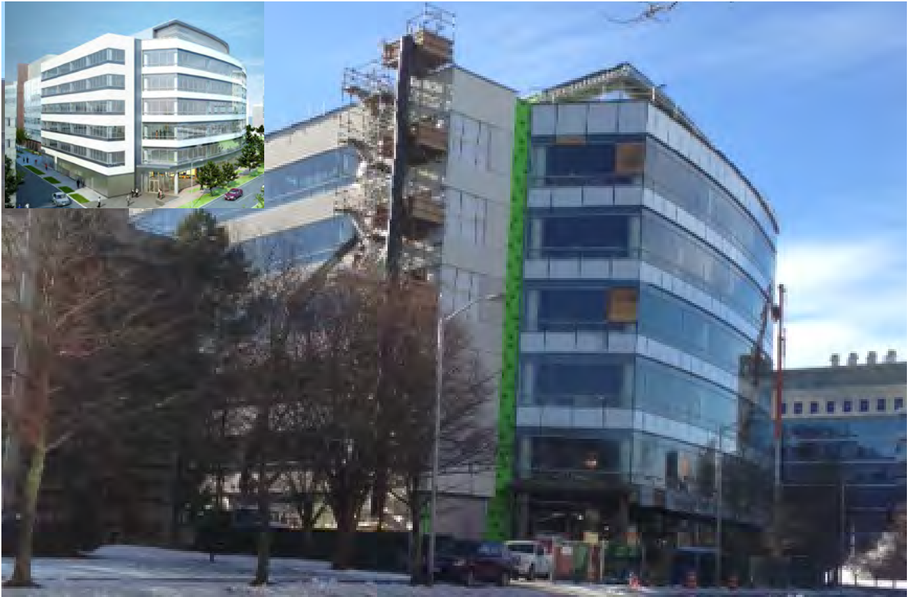
Biogen Expansion (under construction)
