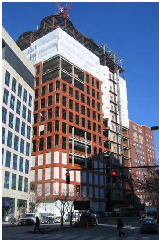
Broad Expansion (under construction)
