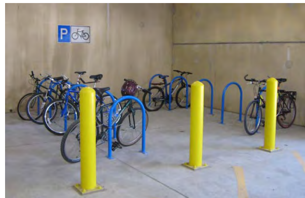
Supportive racks with the benefit of weather protection (above) and garage security with bollards to protect bicycles from cars (below)
