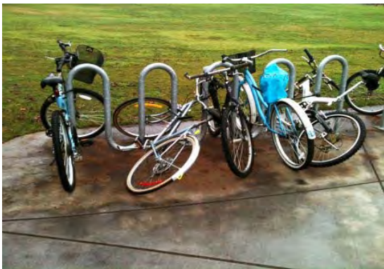
Examples of bicycle racks that do not meet the demand and that do not physically support the bicycles
