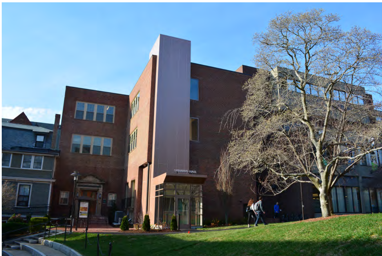
STEBBINS HALL IS NOW ACCESSIBLE FROM THE QUAD VIA A NEW ELEVATOR, PART OF THE SUBSTANTIAL RENOVATIONS TO THE BUILDING.
