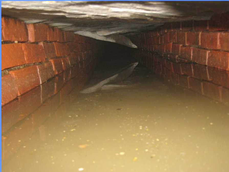
Slate collapse into sewer
