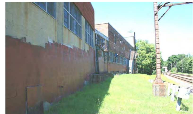
9 Existing Building Looking West on Rail Road Right-of-Way
