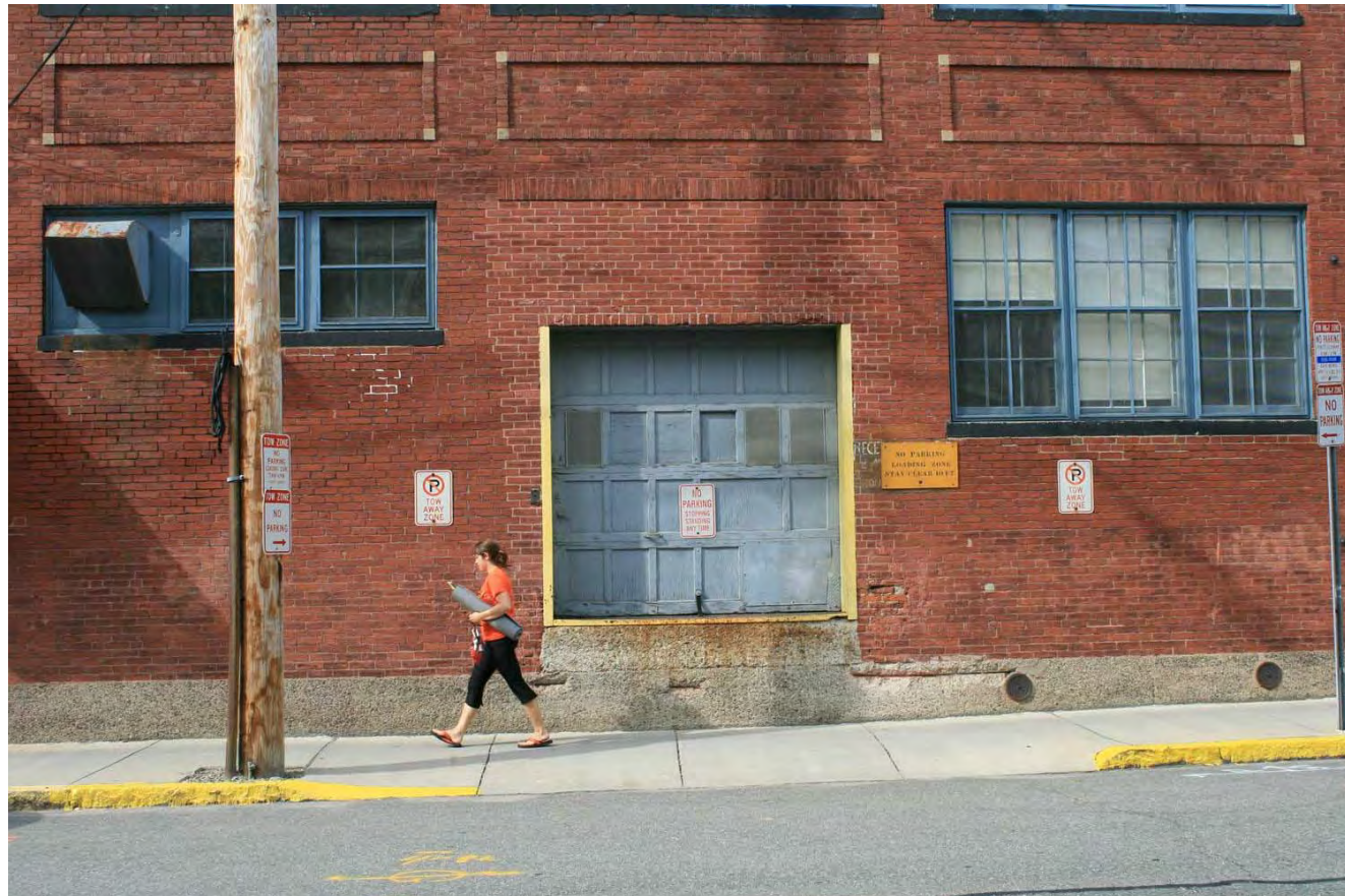
This bay of the building has been adapted over time and no longer bears resemblance to the original 1910 design.
