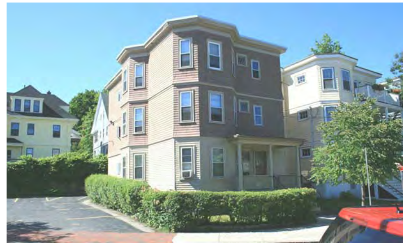
5 General Residential Context Across the Street from Existing Building
