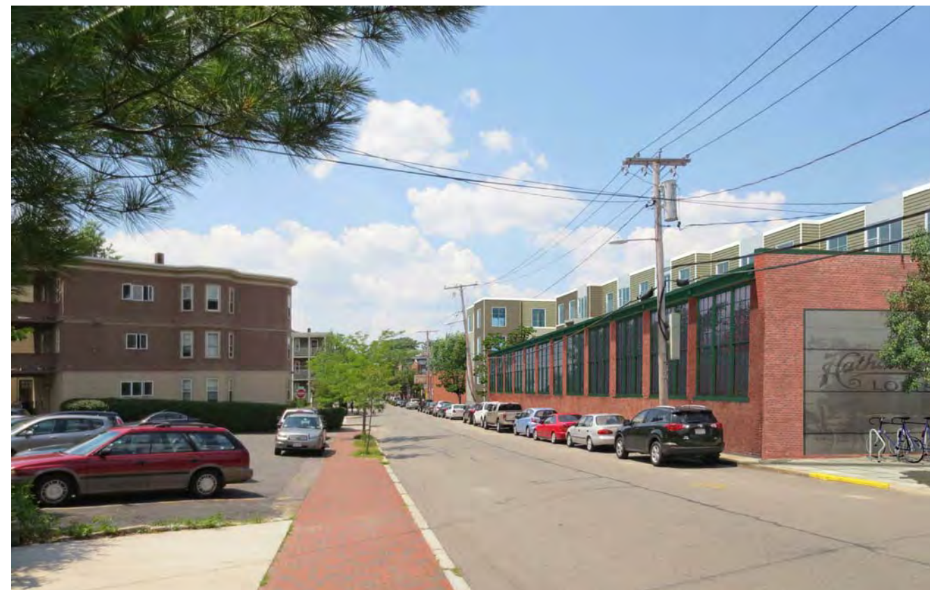
View of Proposed Construction Looking West on Richdale Avenue
