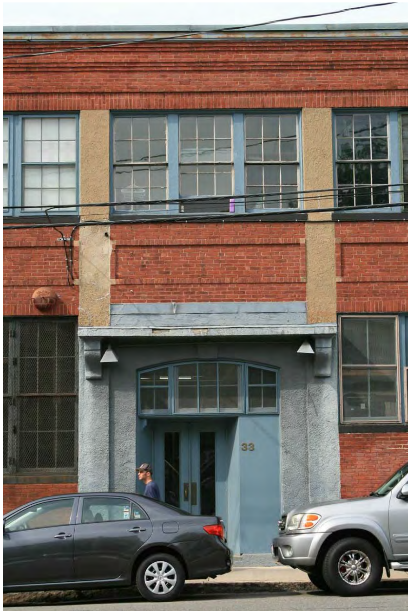
Existing stucco entry is lacking in detail and execution. It is also not handicapped accessible.
