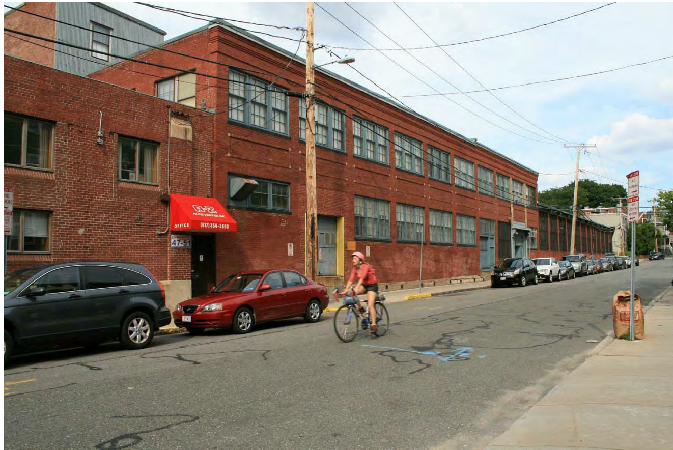
The design proposal is to remove the two story section of the building to create relief and add green space and trees to the streetscape.
