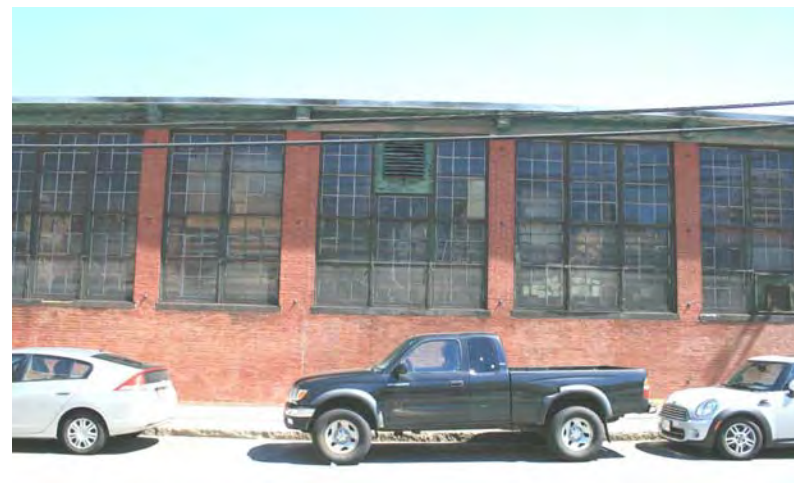
5 Existing Center Bays
