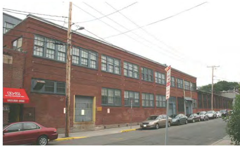
1 Existing Building Looking East on Richdale Avenue
