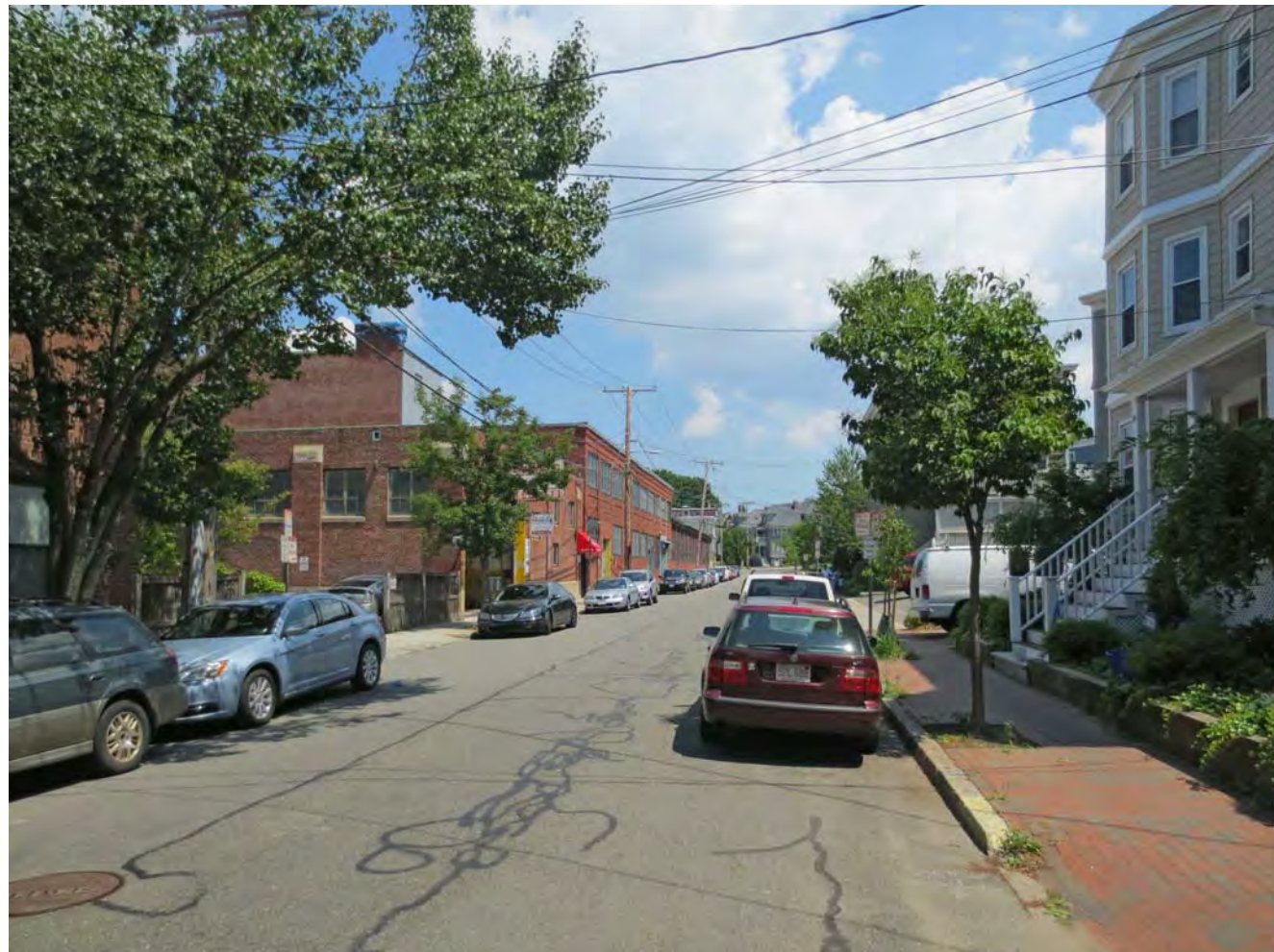
View of Existing Conditions Looking East on Richdale Avenue
