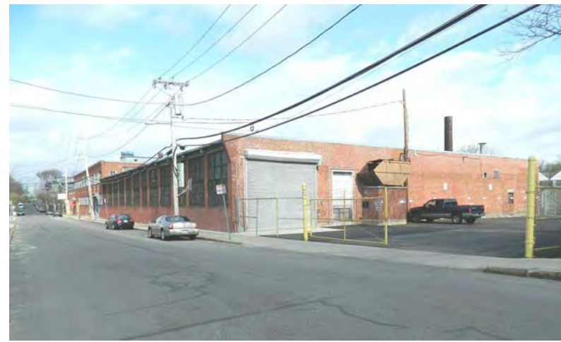
2 Existing Building Looking West on Richdale Avenue
