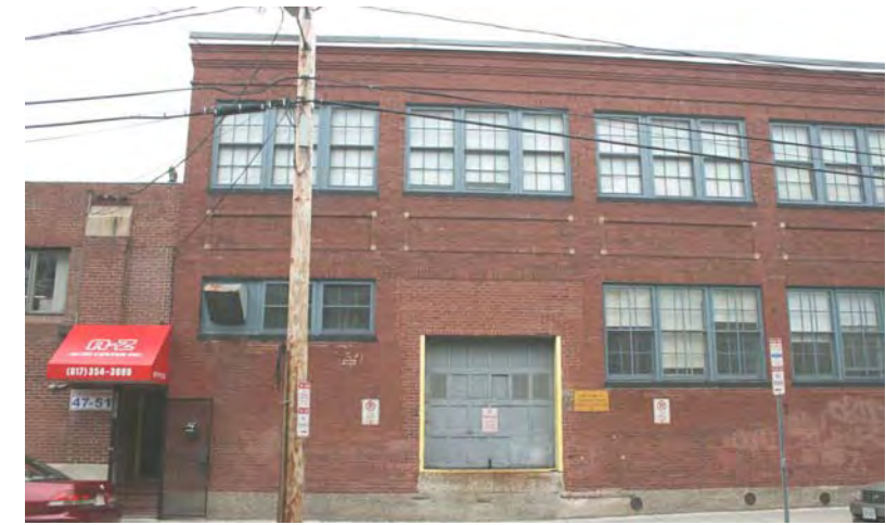
3 Existing Loading Dock
