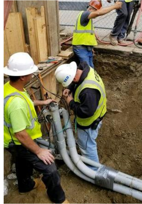
Electrical staff repair an underground conduit.
