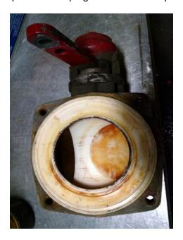
Also discovered was a drain that didn't work. After the motor squad removed the drain, they found debris had clogged the drain. If this stuff is in the drain, it's in your pump and could be plugging your nozzle!
