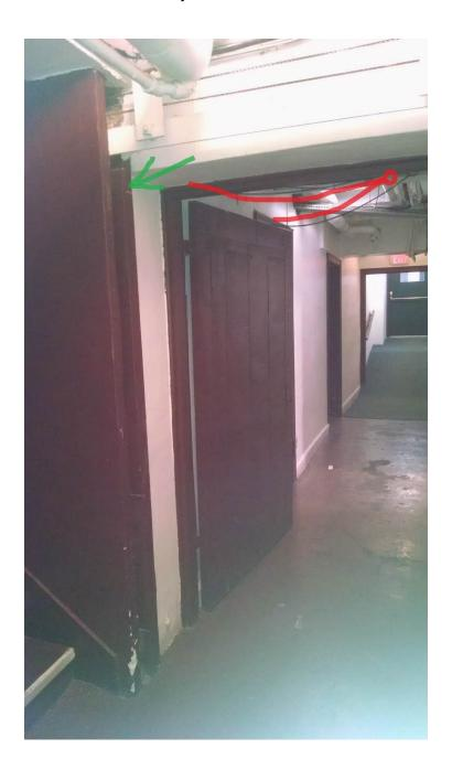
Due to years of neglect, this door would most likely not close even if needed. However, we must always be aware that if doors are properly maintained and operating, they could potentially close behind on crews advancing during firefighting, rescue or ventilation and are heavy and difficult to move should we need a hasty exit. This door on the first floor would most not likely budge due to the paint and dirt buildup, or lack of maintenance on the door roller.
