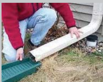
A. Downspout disconnected. Elbow capped.
