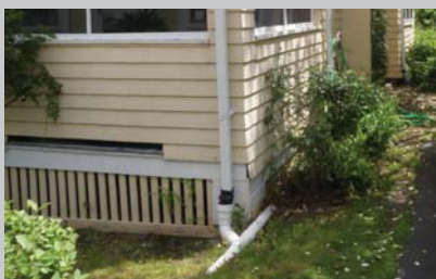
Downspout/roof leader going into basement foundation
