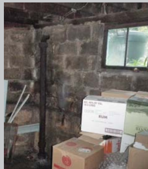
Downspout/roof leader going into basement foundation
