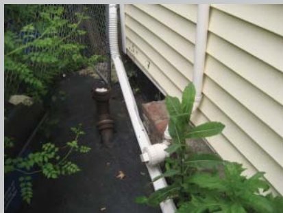
A. Downspout disconnected. Elbow capped.
