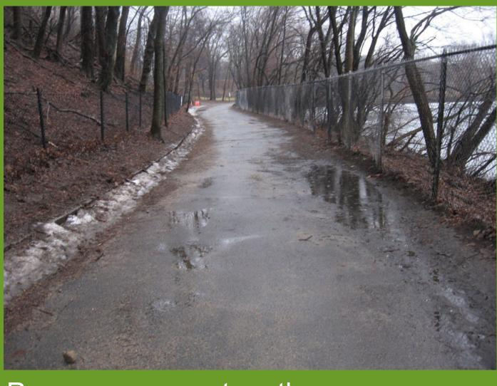
Porous pavement on the Perimeter Road will improve drainage
