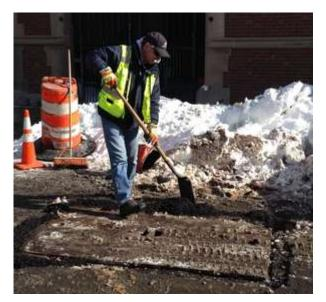
DPW staff secure a roadway steel plate by placing asphalt around the edges
