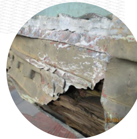
replacement of perimeter dentilled fascia to 1927 details (where necessary)
