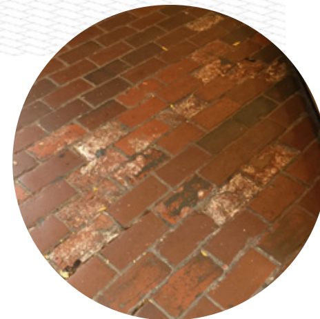
address MAAB compliant brick floor
