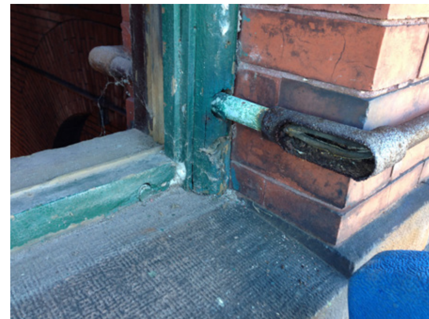
The original window frames at the upper clerestory provided evidence of the original frame design and brickmold profiles.
