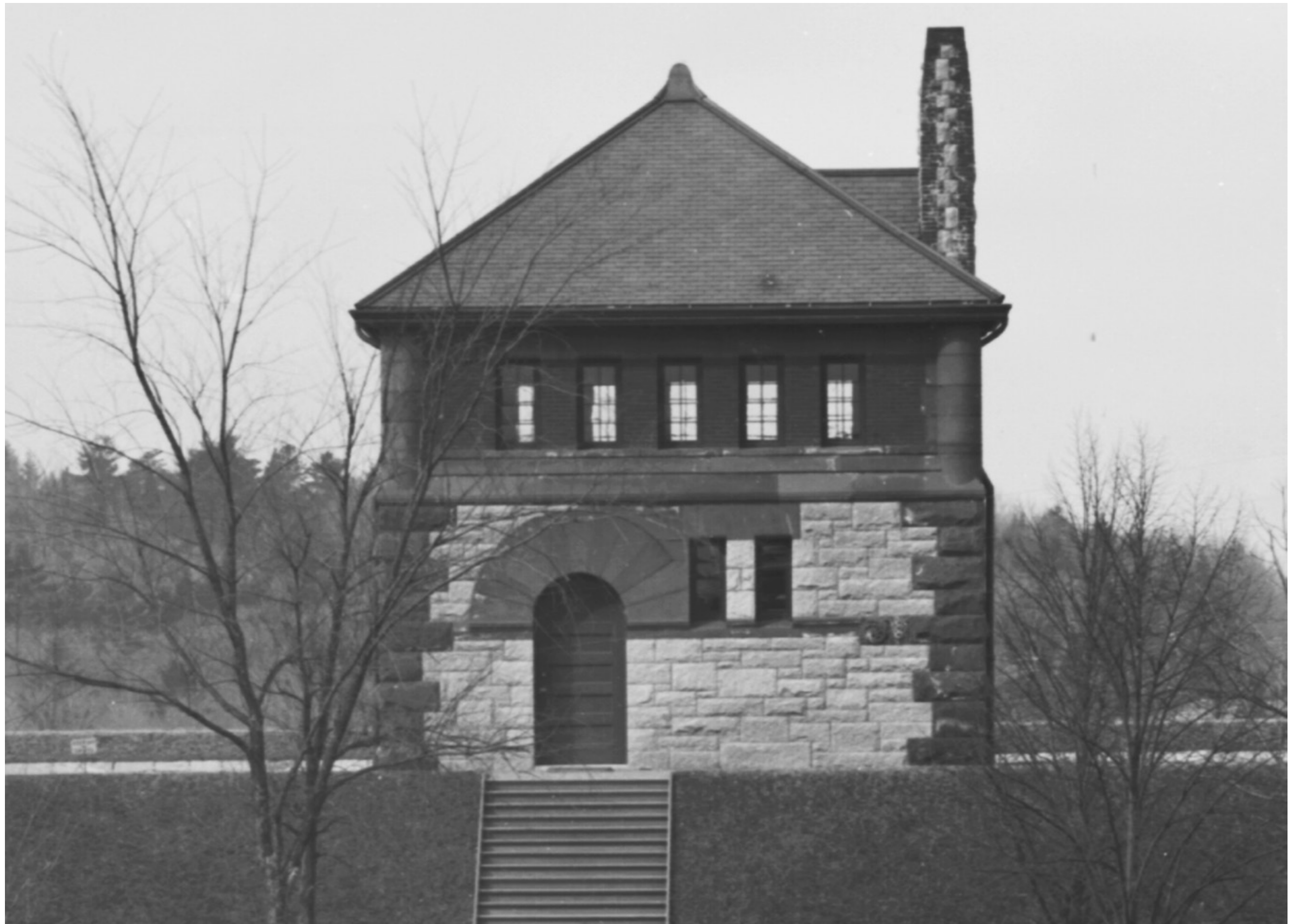
Historic photo - view southwest reservoir in-use. Historic photos like this along with remnants of the original windows and door wood profiles were analyzed during the design phase to reconstruct the windows doors & louvers to their original appearance.
