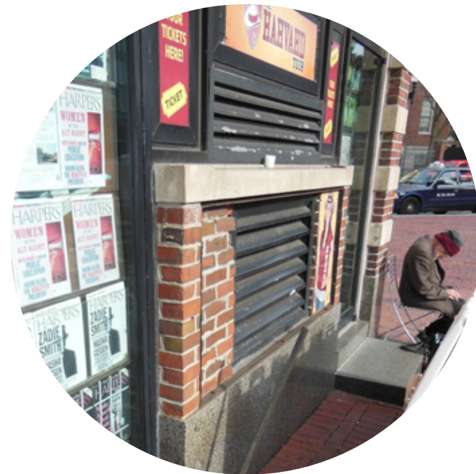
removal of vents along south elevation
