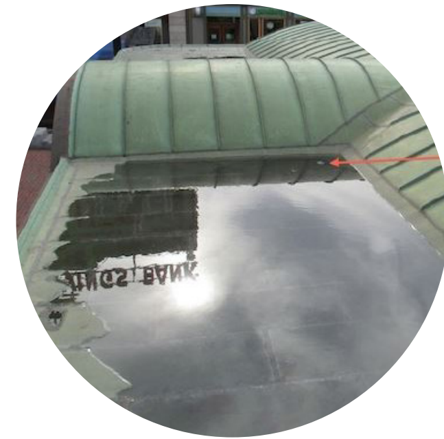
replacement of standing seam copper roof & allow for thermo dynamic movement
