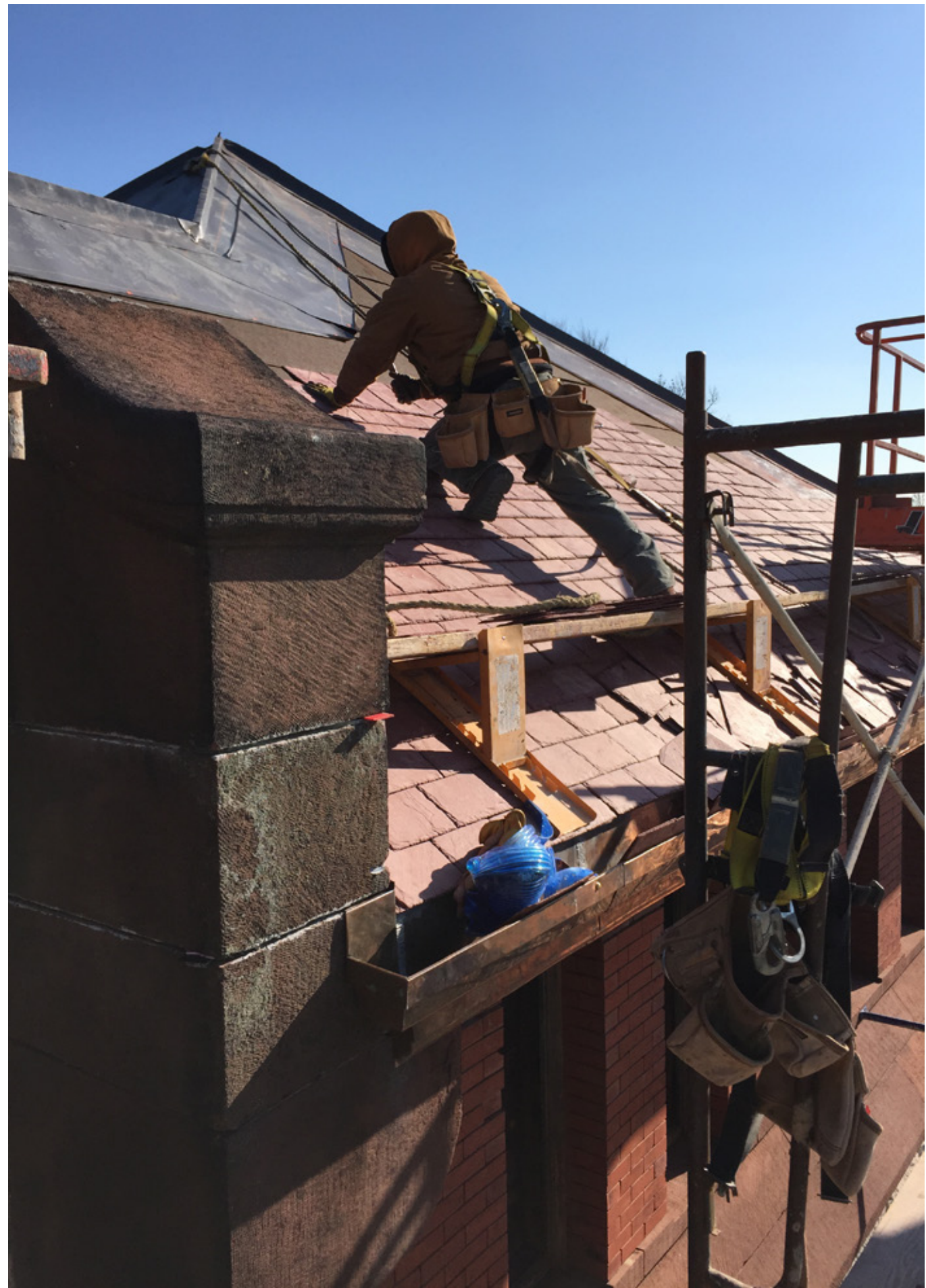
Slate roof installation. Design team matched color, size and installation methods.
