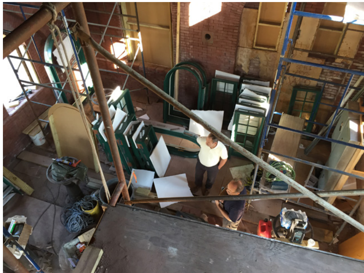
Mock-ups and installation of the Gatehouse windows.
