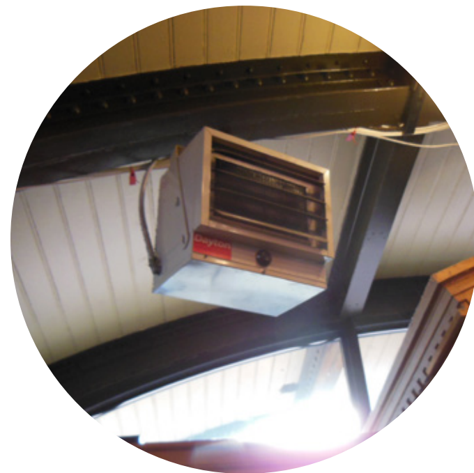
removal of all interior & exterior heating and cooling units for redesign of systems for greater efficiency
