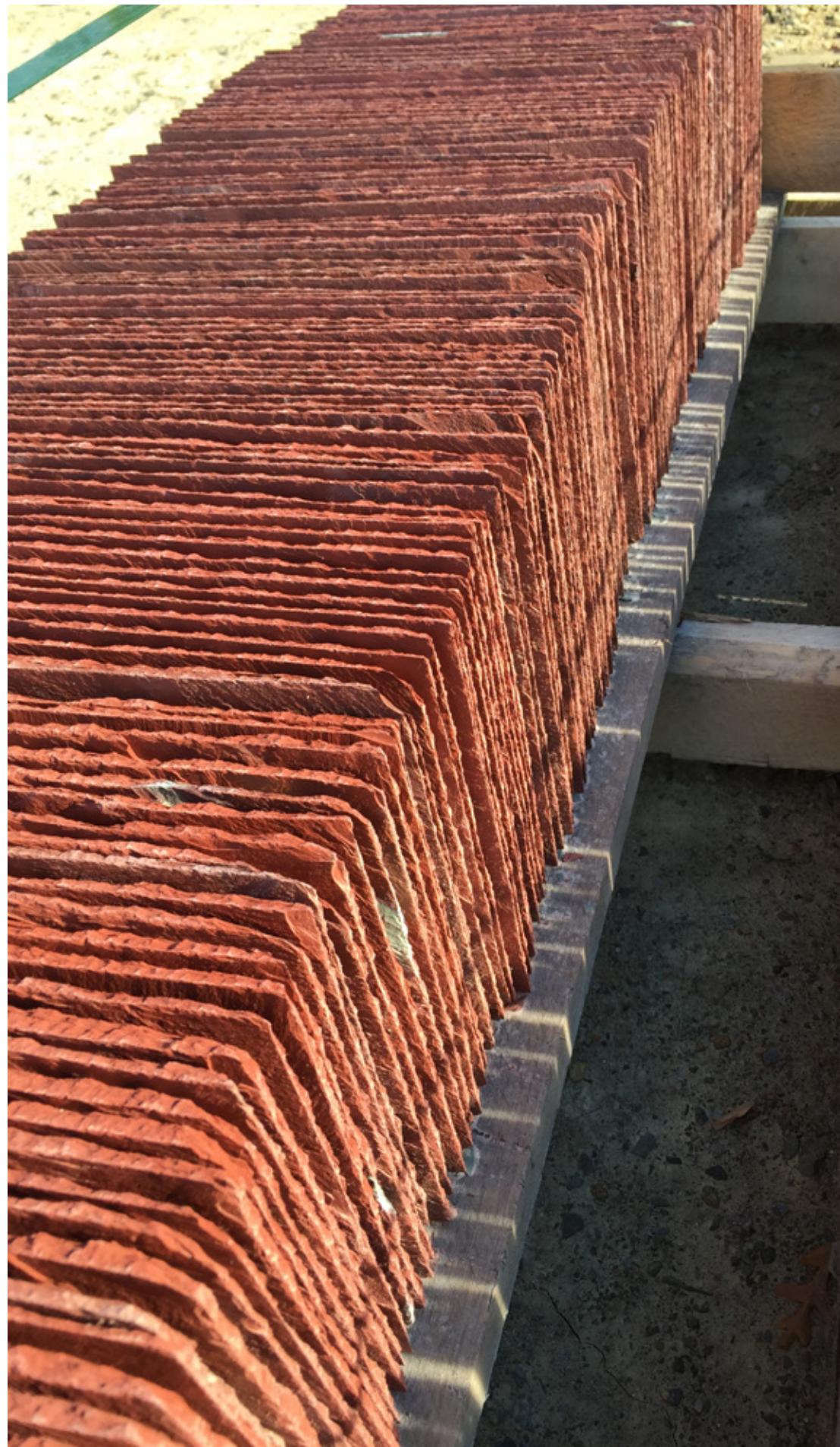
New slate roof tiles
