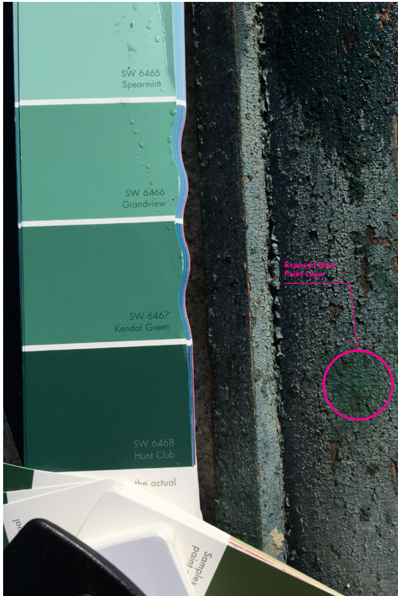
Original painted wood base layer revealed with paint swatch comparison for color match.
