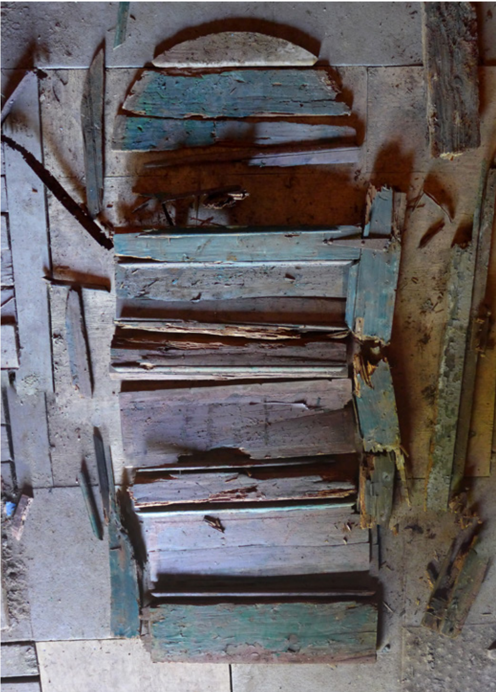
Original door pieces salvaged from bottom of gate chamber re-assembled
