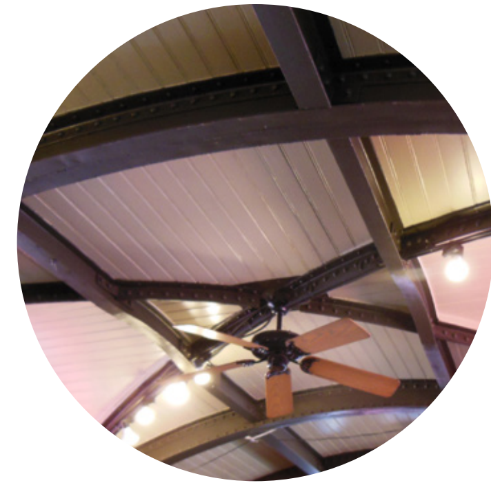
preserve exposed wood beadboard & riveted iron structure
