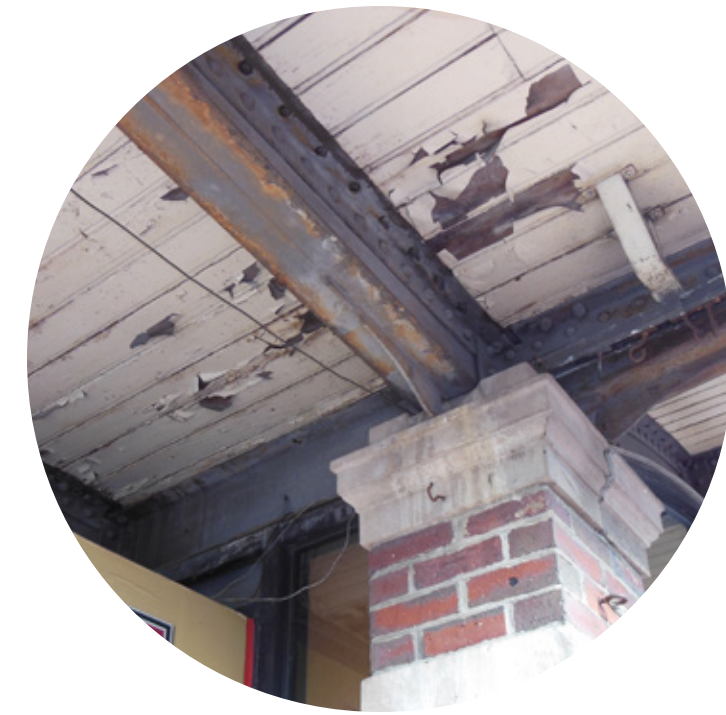
restoration / replacement of exposed beadboard
