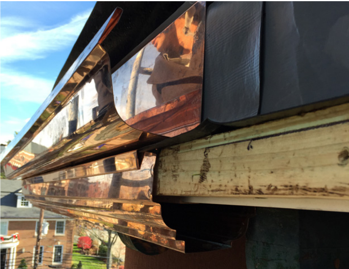
Recreated copper gutter and flashing details to match profiles and installation.
