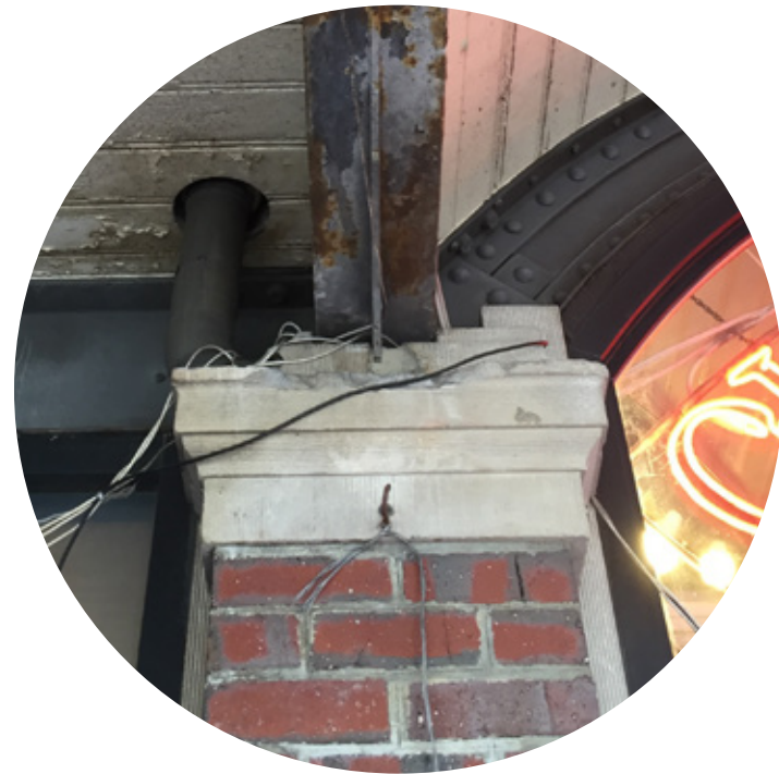
repointing of mortar joints to maintain color, texture and profile of original joints
