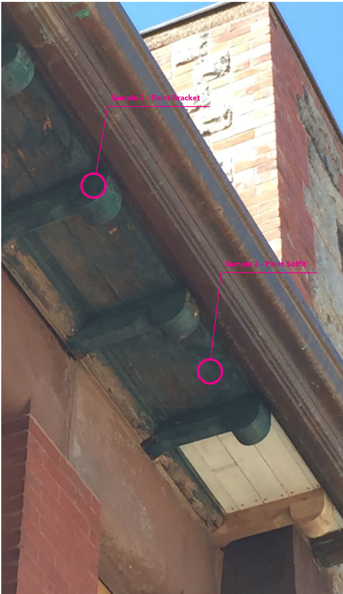
Replaced wood soffit and bracket to match existing.
