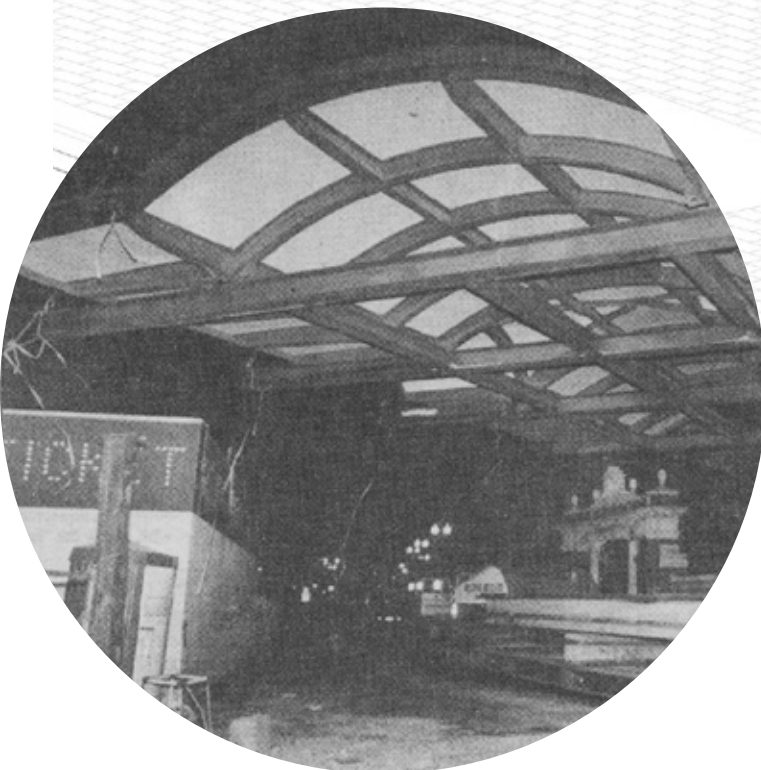
re-installation of original kiosk roof - 1983
