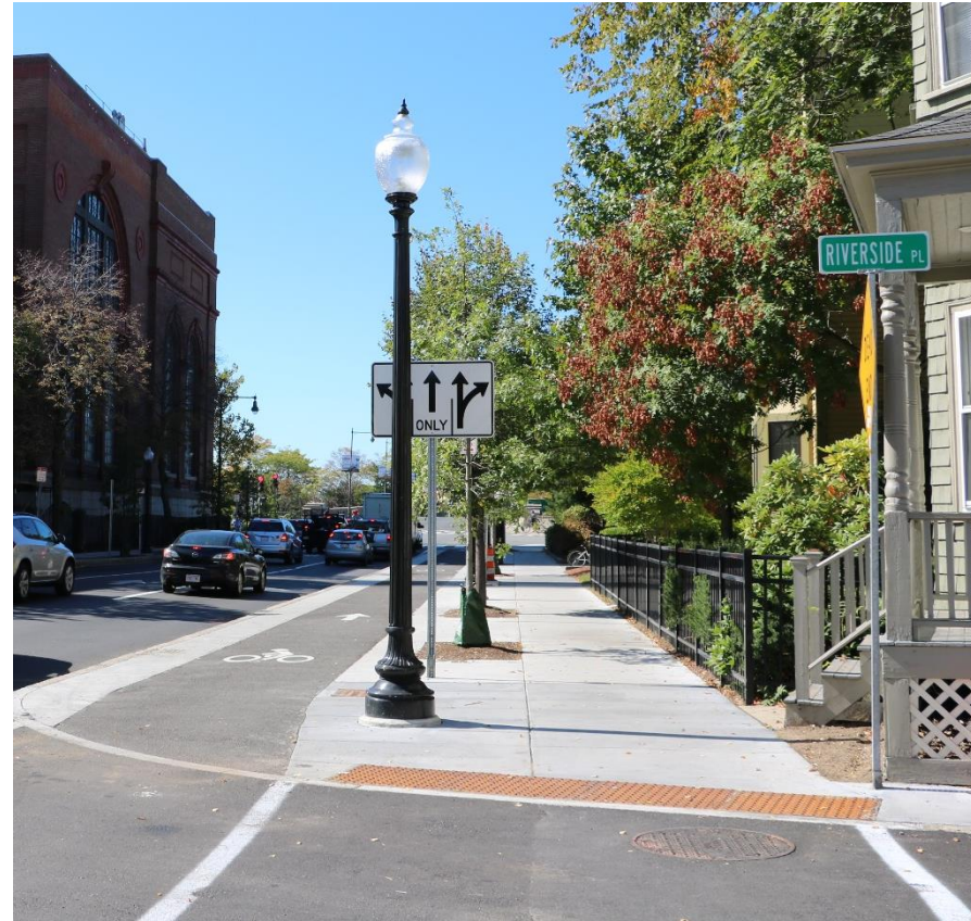
Pedestrian Lighting ( Western Ave )
