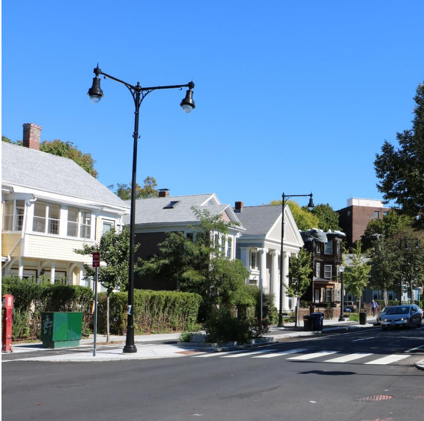
Roadway Lighting ( Western Ave )
