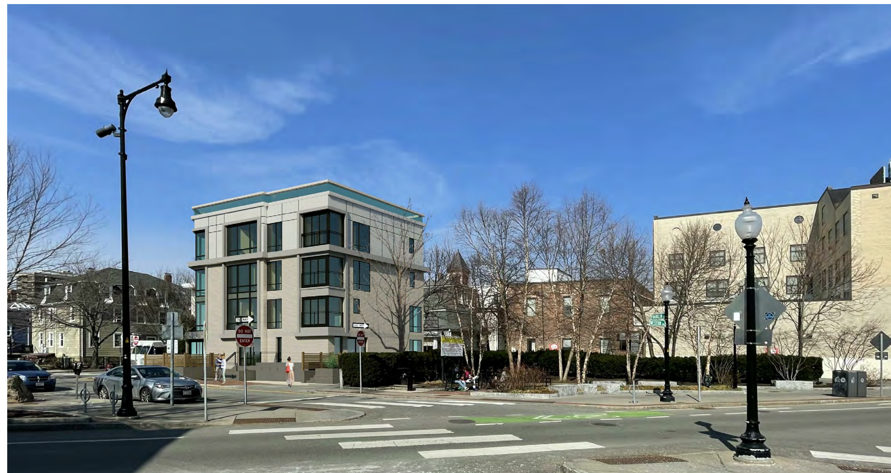
VIEW AT WESTERN AVE - PREVIOUS
