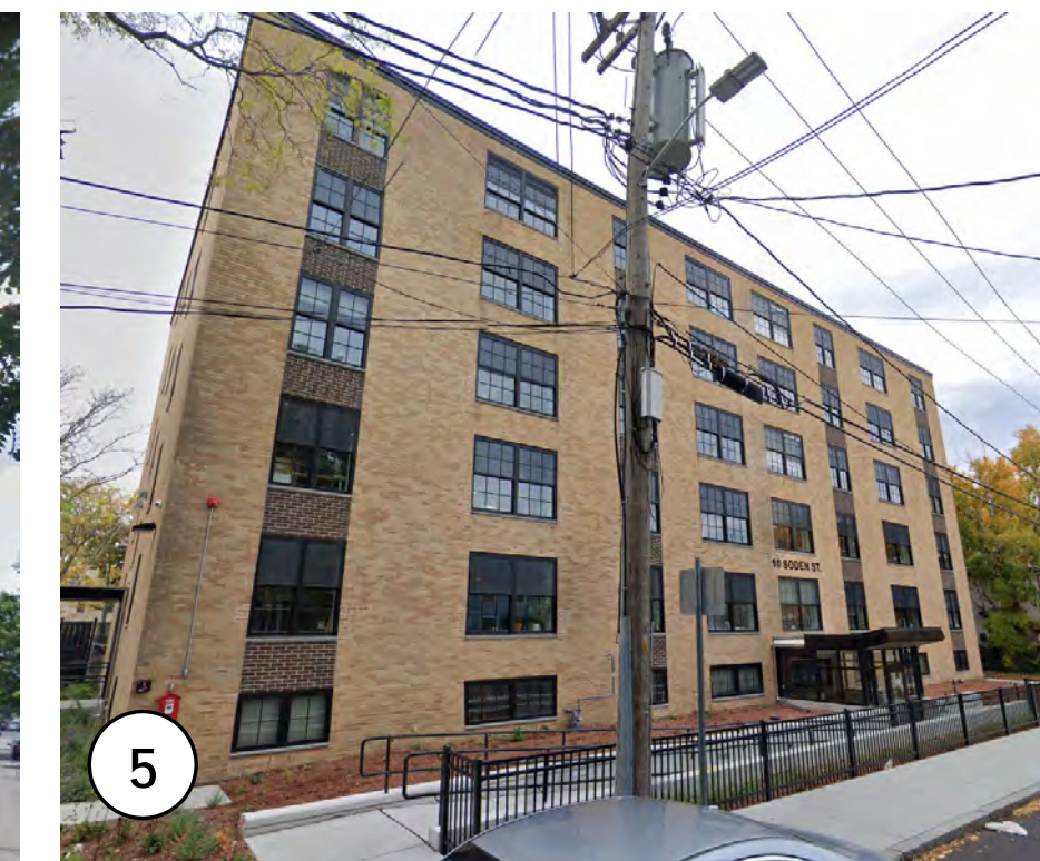
5 10 SODEN STREET 5 1/2 STORIES RESIDENTIAL BUILDING
