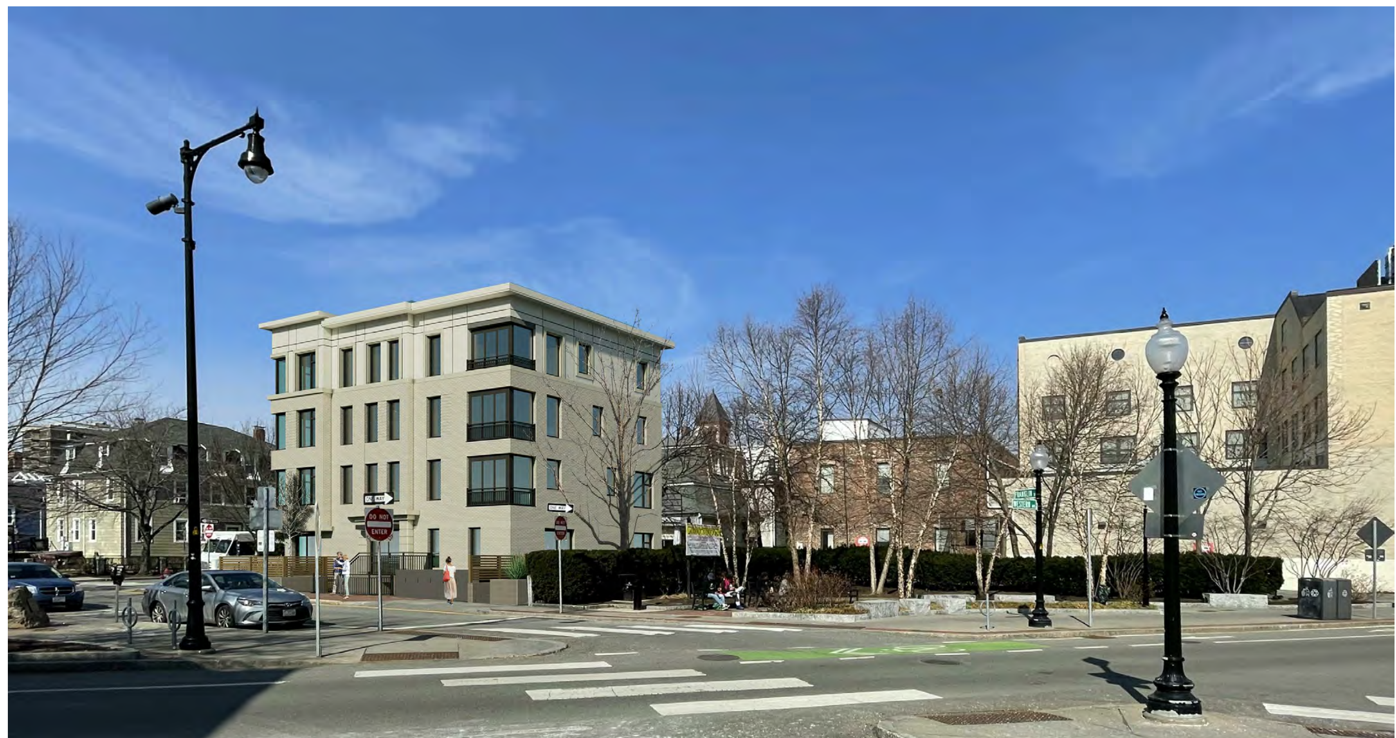
VIEW AT WESTERN AVE - CURRENT
