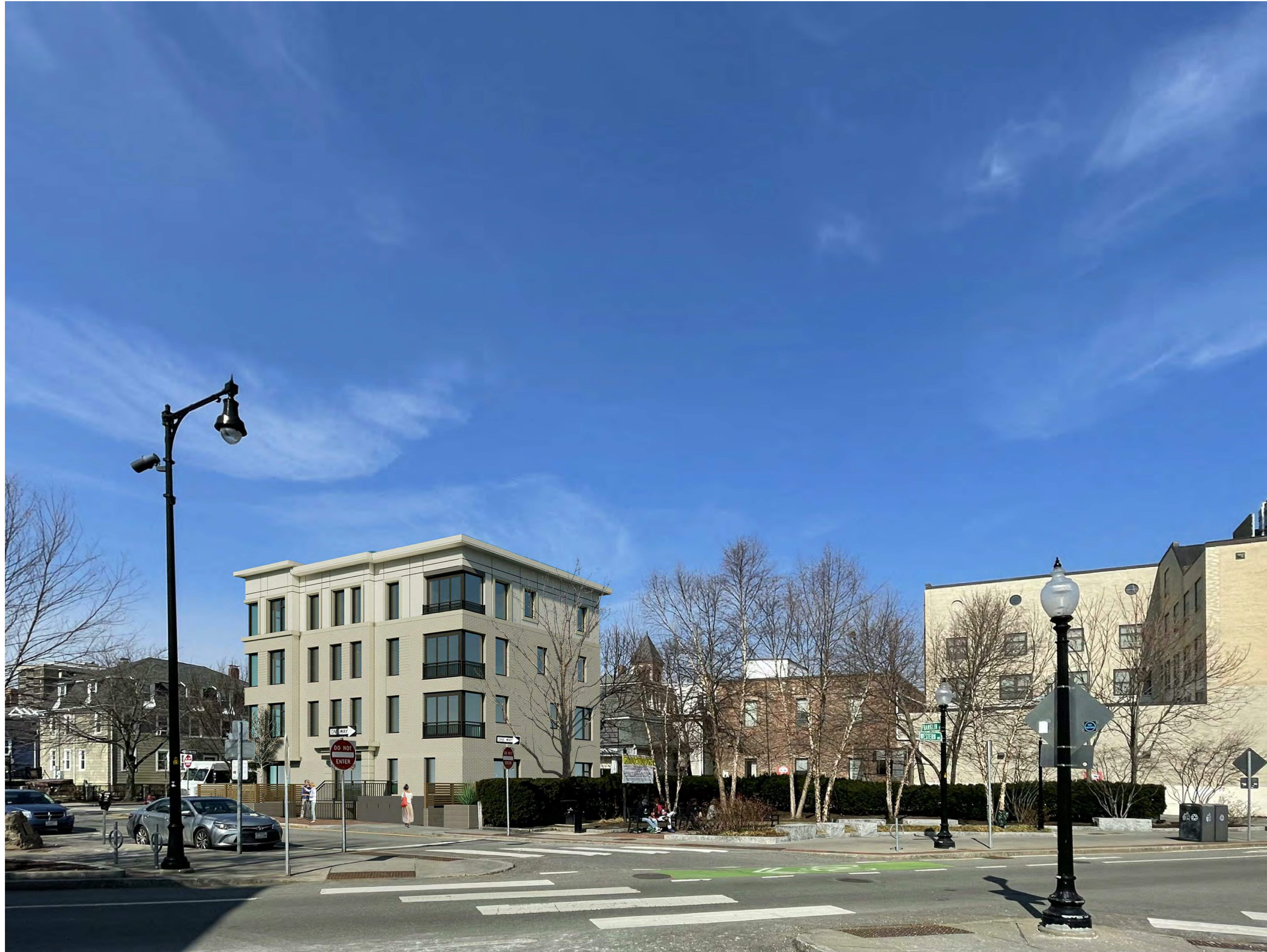
VIEW AT WESTERN AVENUE
