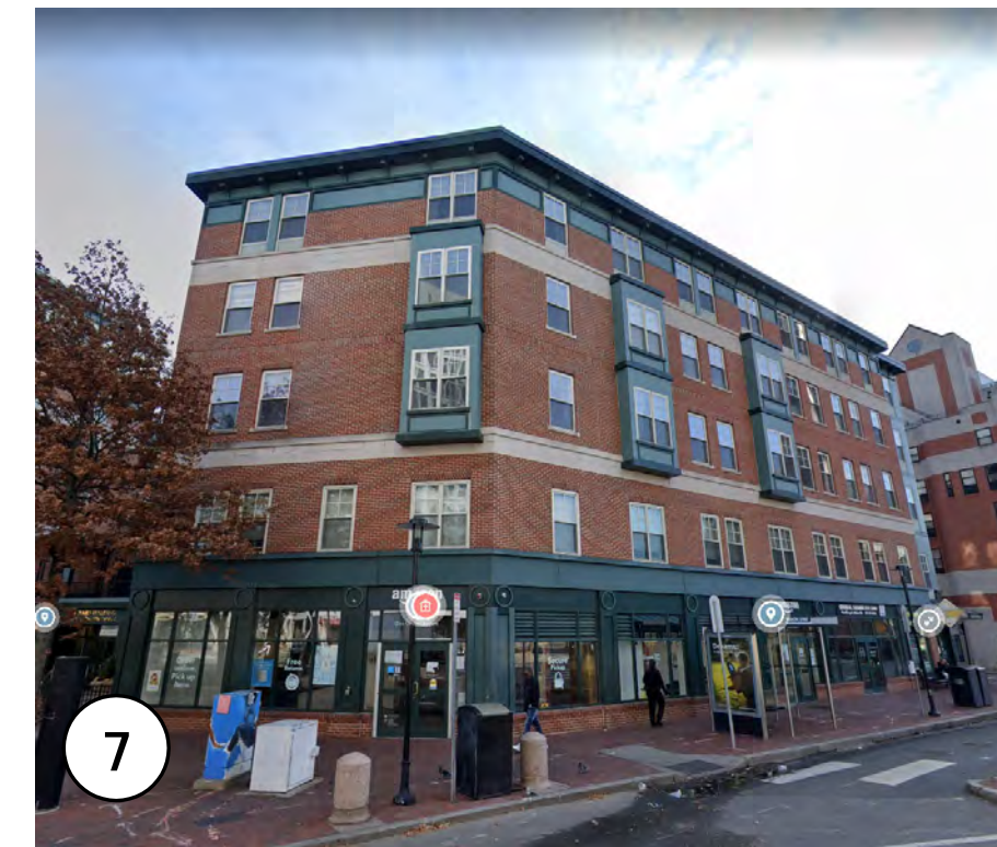
7 1 CENTRAL SQUARE 5 STORIES MIXED-USE BUILDING
