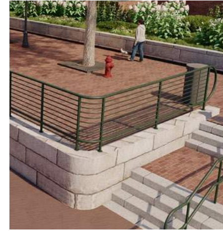
NEW HANDRAIL AND GUARDRAILS WHERE REQUIRED
