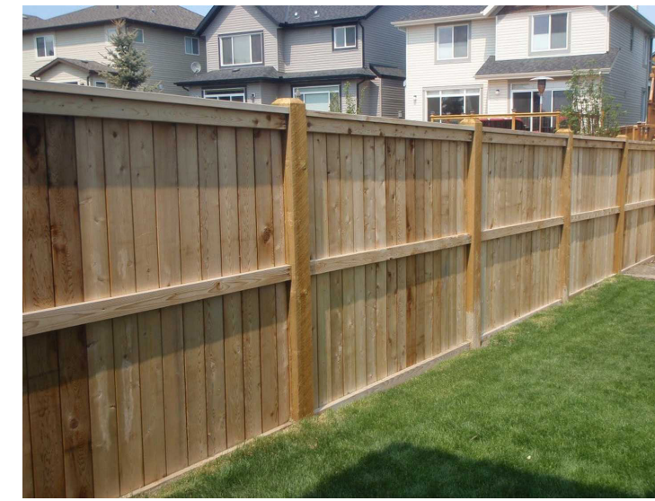
Wood Board Fence
