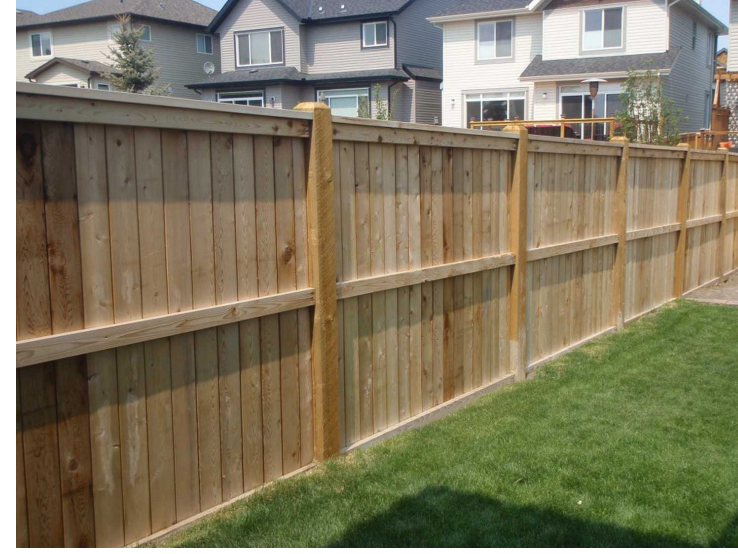
Wood Board Fence
