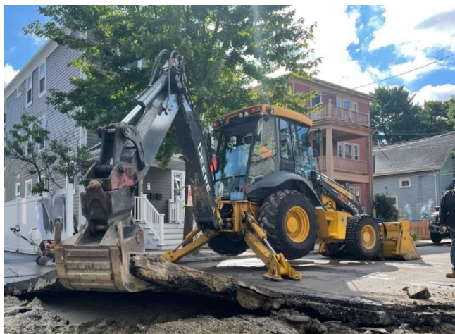
Repairing a street
