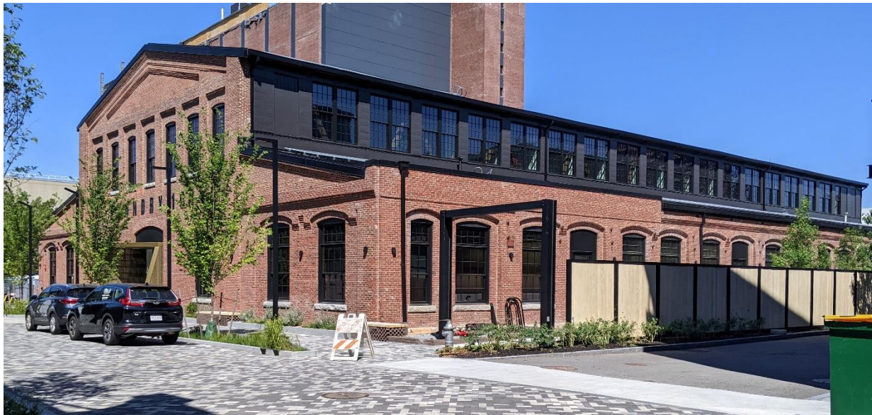
The newly renovated Foundry building
