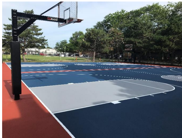
Renovated basketball court at Kennedy Longfellow School.
